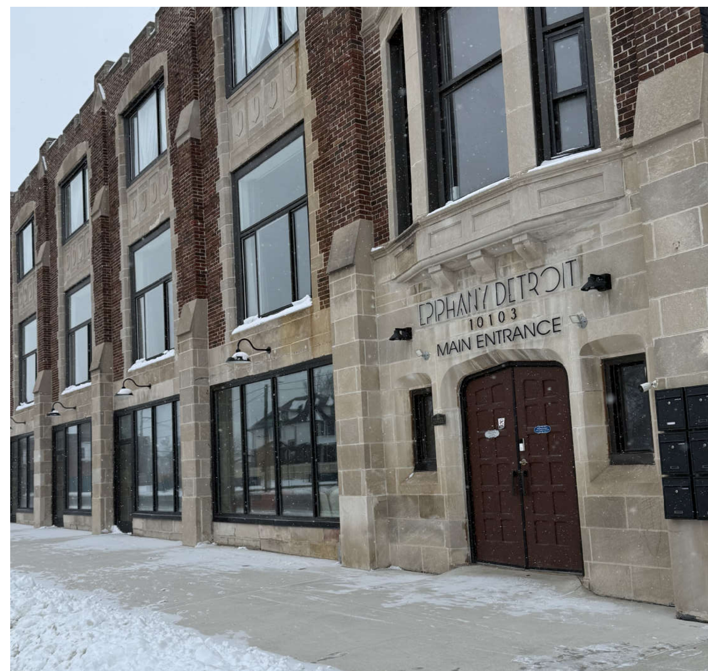
WALL LIGHT ABOVE RIGHT OF WAY
