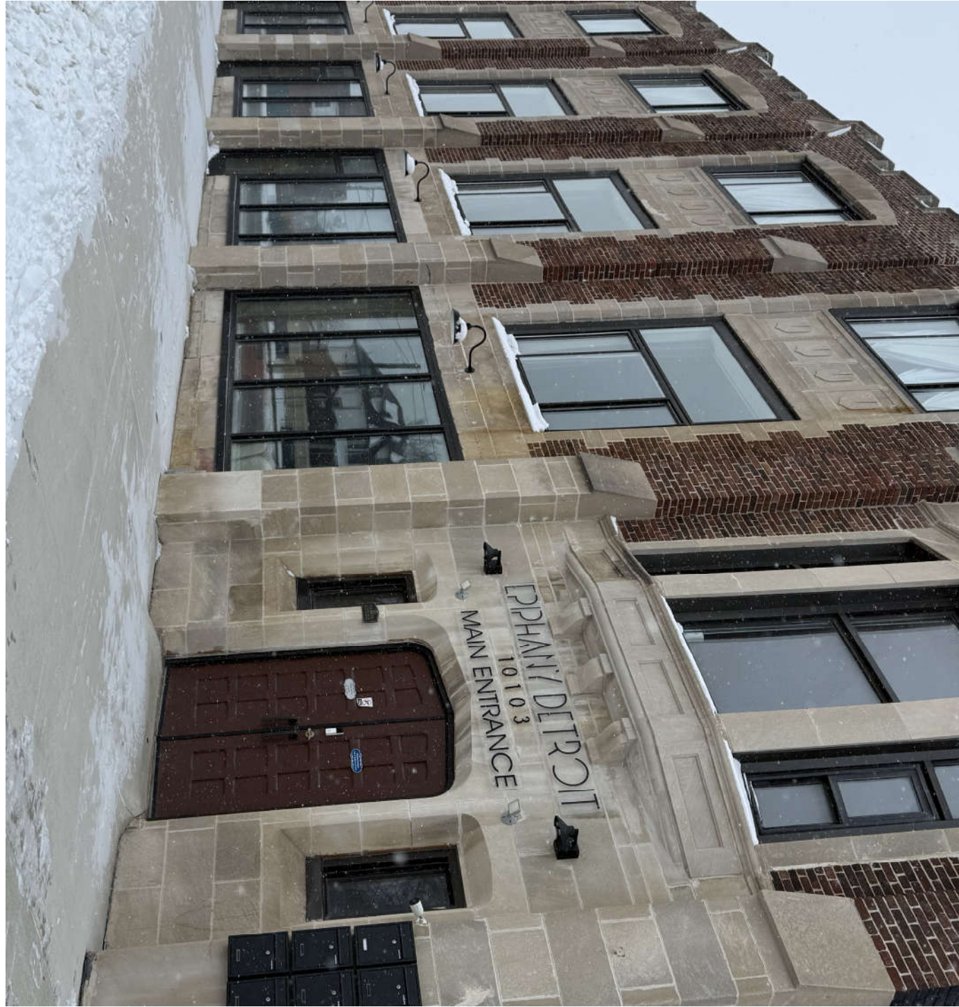
WALL LIGHT ABOVE RIGHT OF WAY
