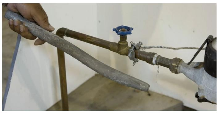
Example of the lead pipe being held up against the copper that has been installed.
