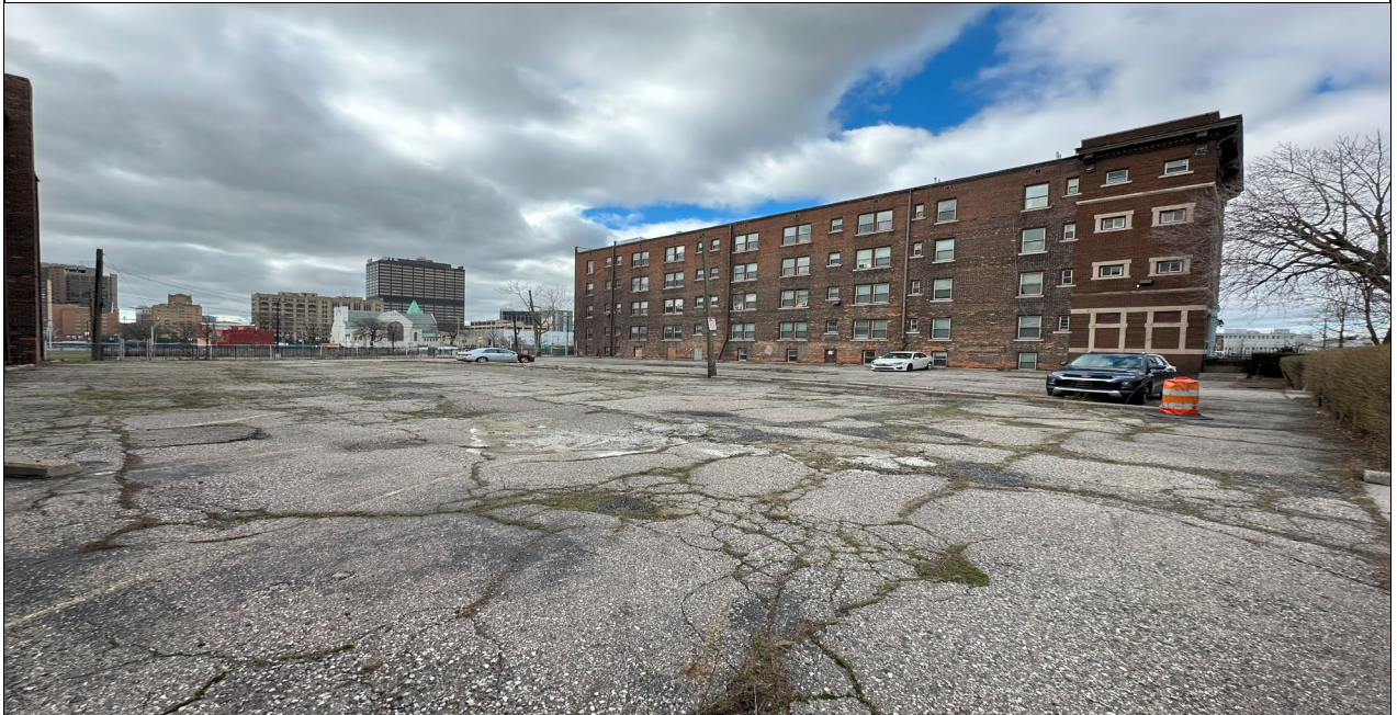
Photograph 8. Northeast side of 489 Henry Street, facing southwest.
