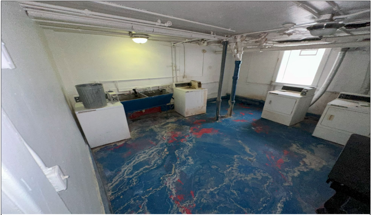
Photograph 19. 489 Henry Street Parcel: Laundry room.
