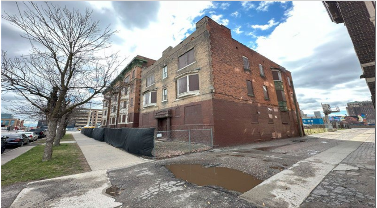
Photograph 5. Overview of 427 Henry St. and 2467 Cass Ave., facing east.
