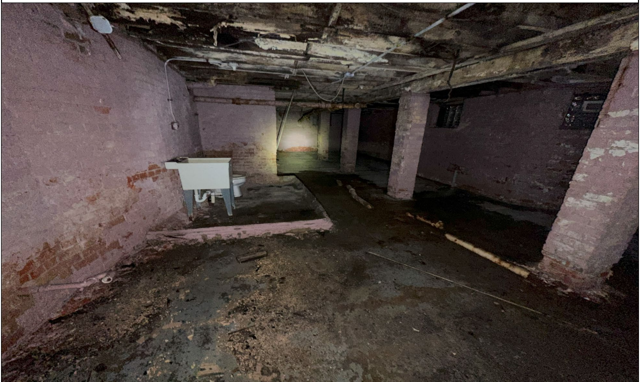
Photograph 16. 427 Henry Street Parcel: Typical basement area.
