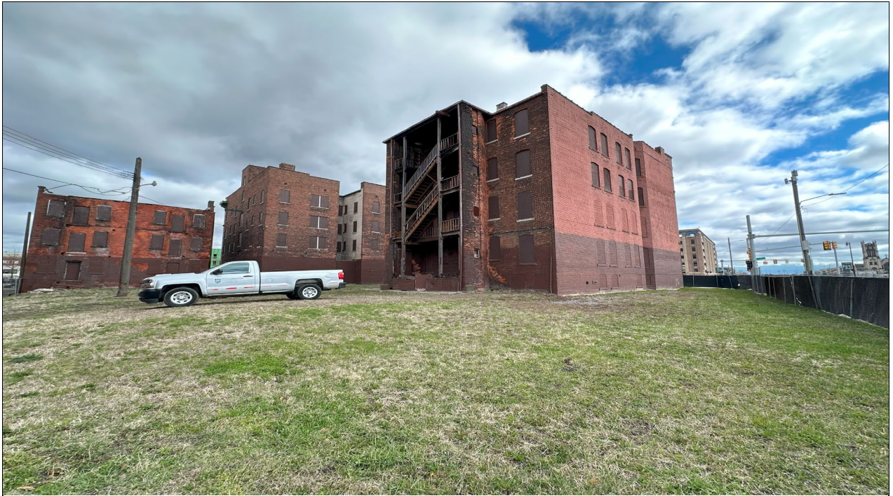
Photograph 1. 2445 Cass Avenue parcel, facing north.
