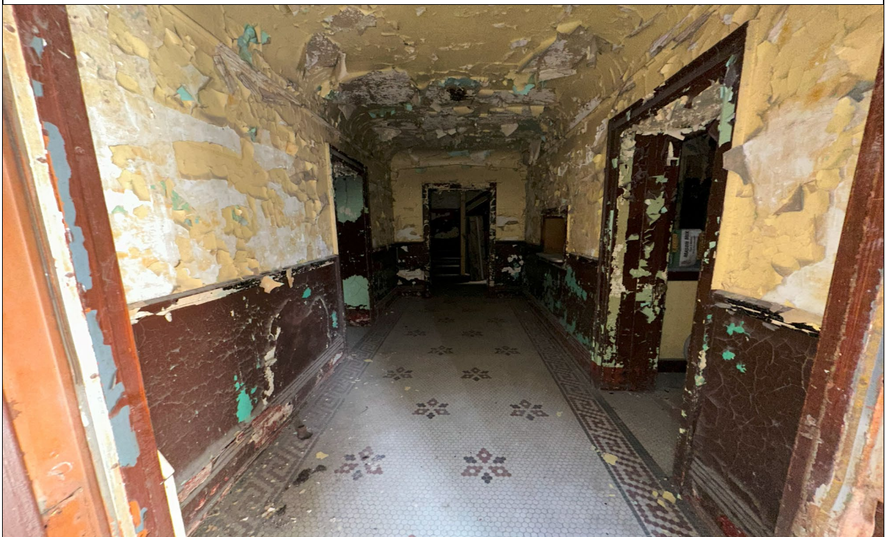
Photograph 12. 2447 Cass Avenue Parcel: Typical hallway.
