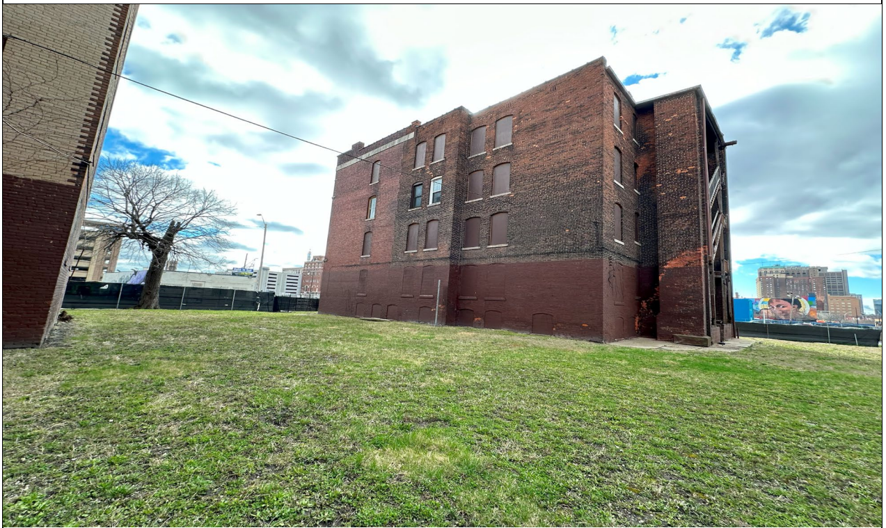
Photograph 4. East side of 2457 Cass Avenue parcel, facing west.
