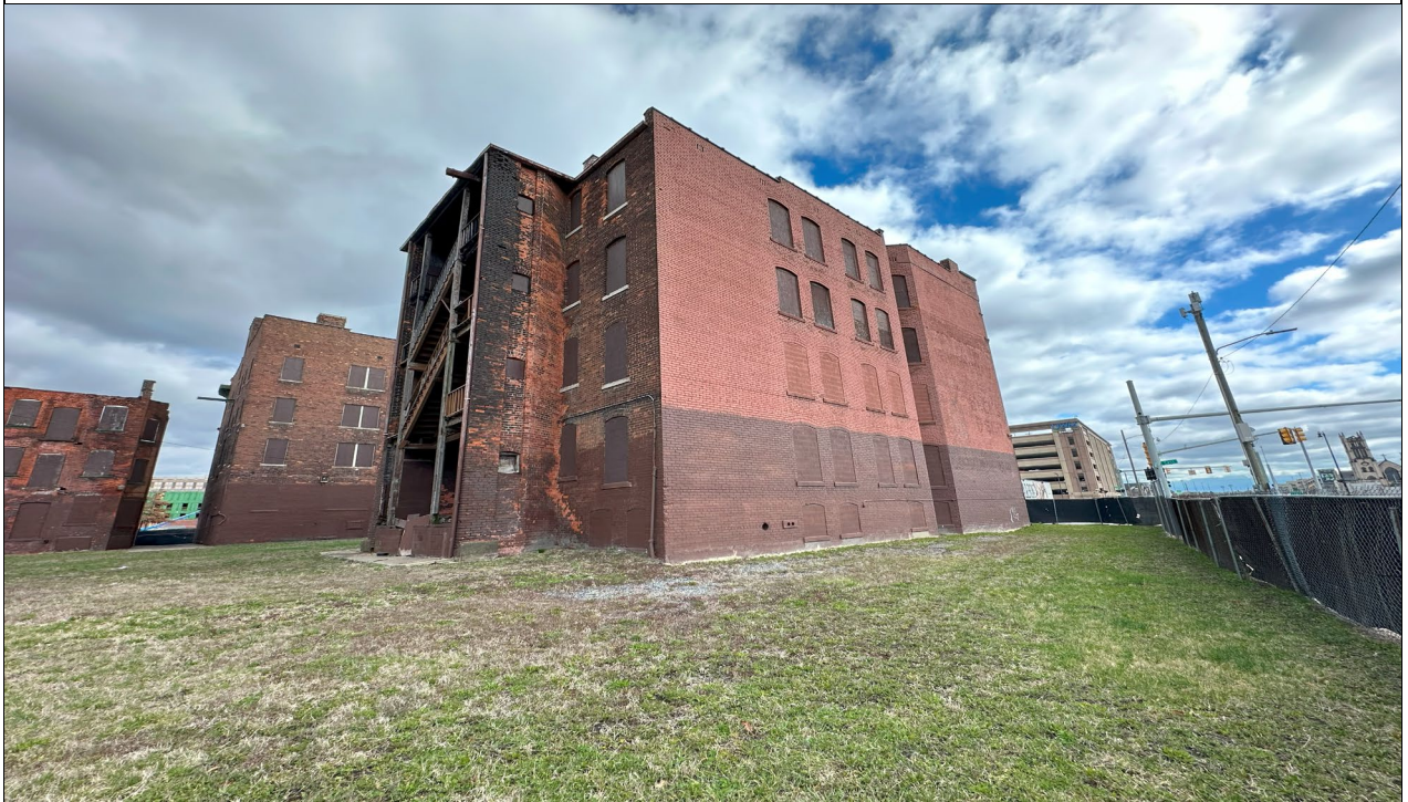
Photograph 2. Southeast corner of 2447 Cass Avenue parcel, facing northwest.
