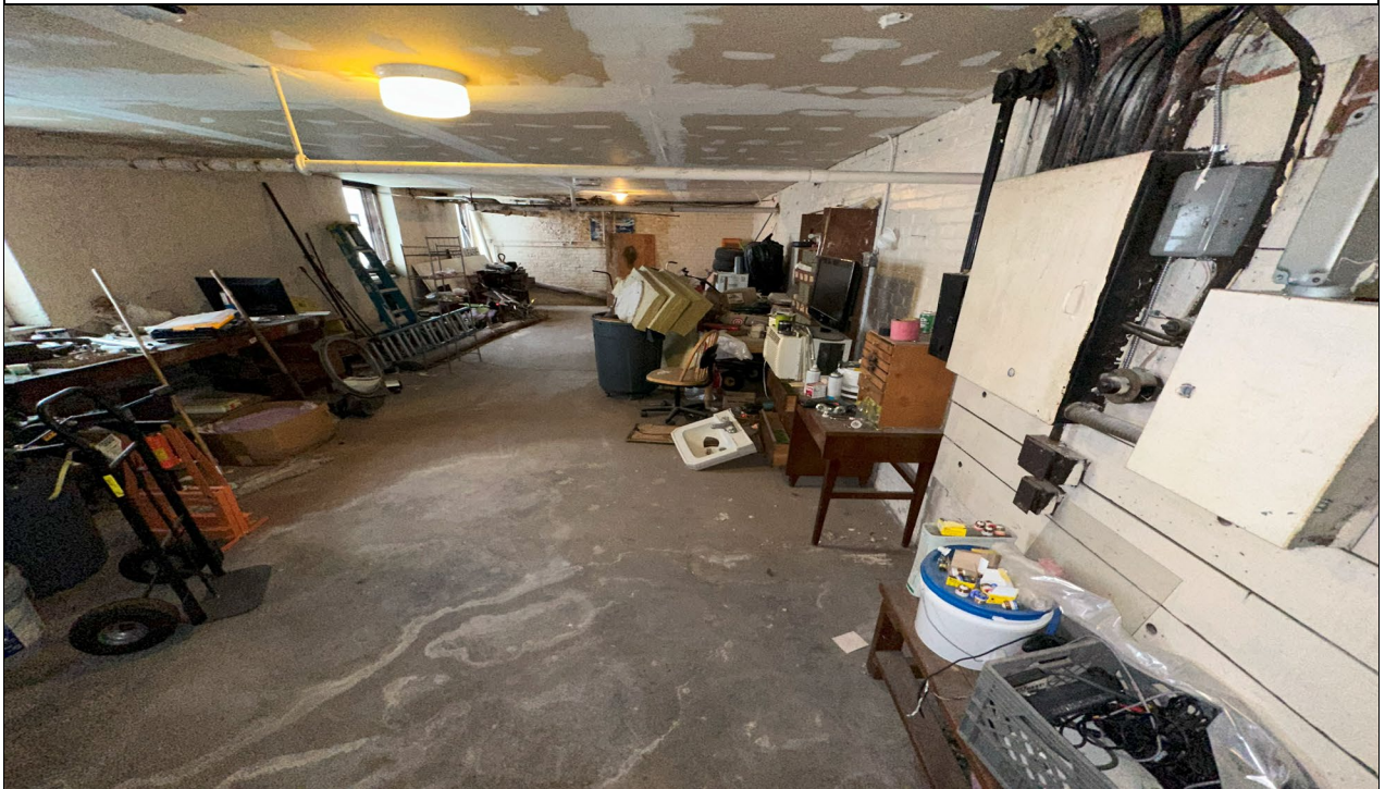
Photograph 18. 489 Henry Street Parcel: Storage room.
