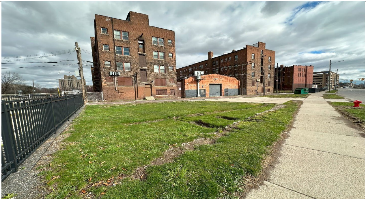
Photograph 10. Western extent of 412, 434 & 450 W. Fisher Street parcels, facing northeast.
