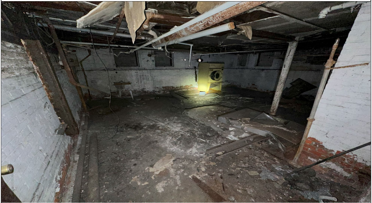
Photograph 14. 2447 Cass Avenue Parcel: Typical basement area.
