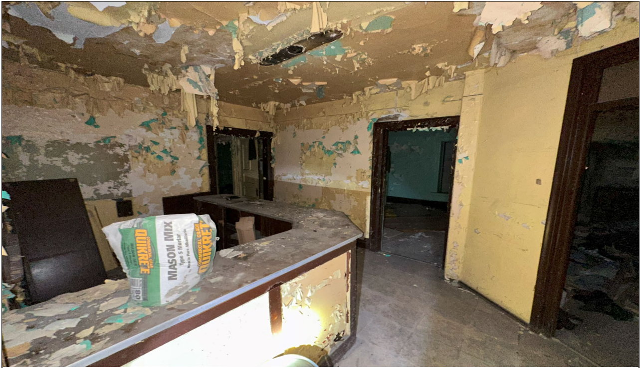
Photograph 11. 2447 Cass Avenue Parcel: Lobby area.
