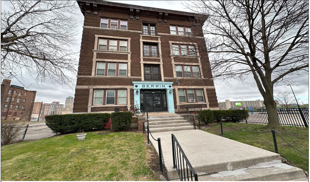
Photograph 7. North exterior of 489 Henry Street, facing south.
