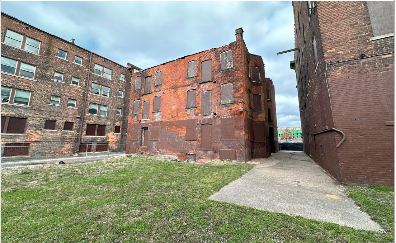
Photograph 6. South side of 427 Henry Street, facing north.
