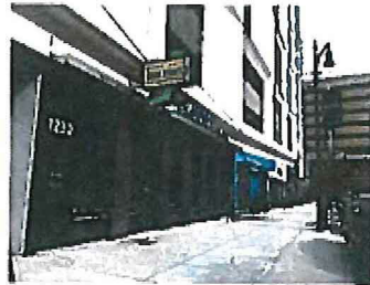
3 | EXISTING CONDITIONS SOUTHEAST VIEW
