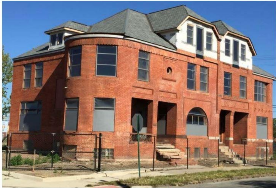
Existing Southwest Corner
