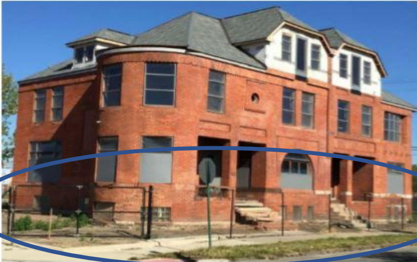
EXISTING SOUTHWEST CORNER
