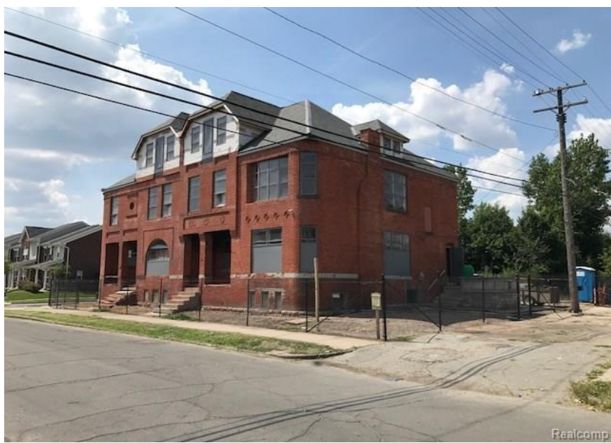
Existing Southeast Corner
