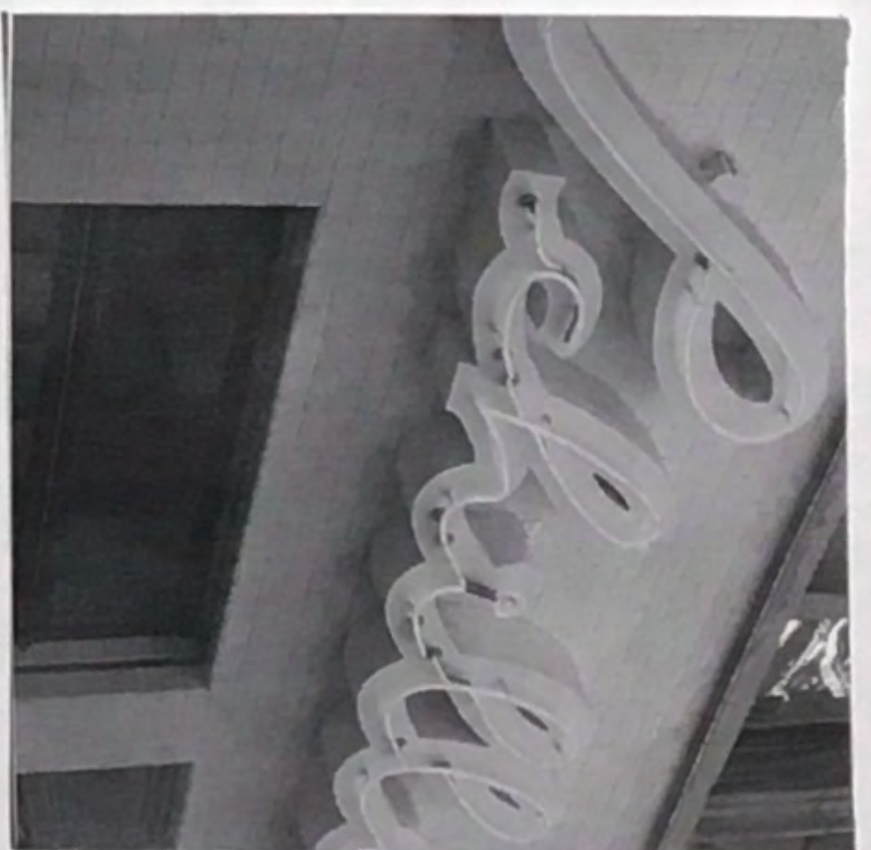
SIGNAGE: NEON MOUNTED OVER DIMENSIONAL LETTERS
