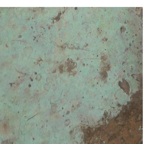
PATINA COPPER FINISH ON ENTRY DOOR
