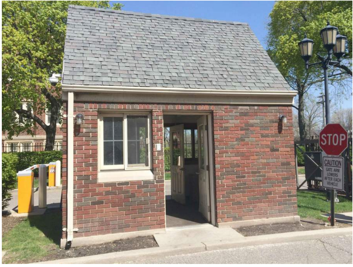
REFERENCE PHOTO 02 EXISTING GATE HOUSE
