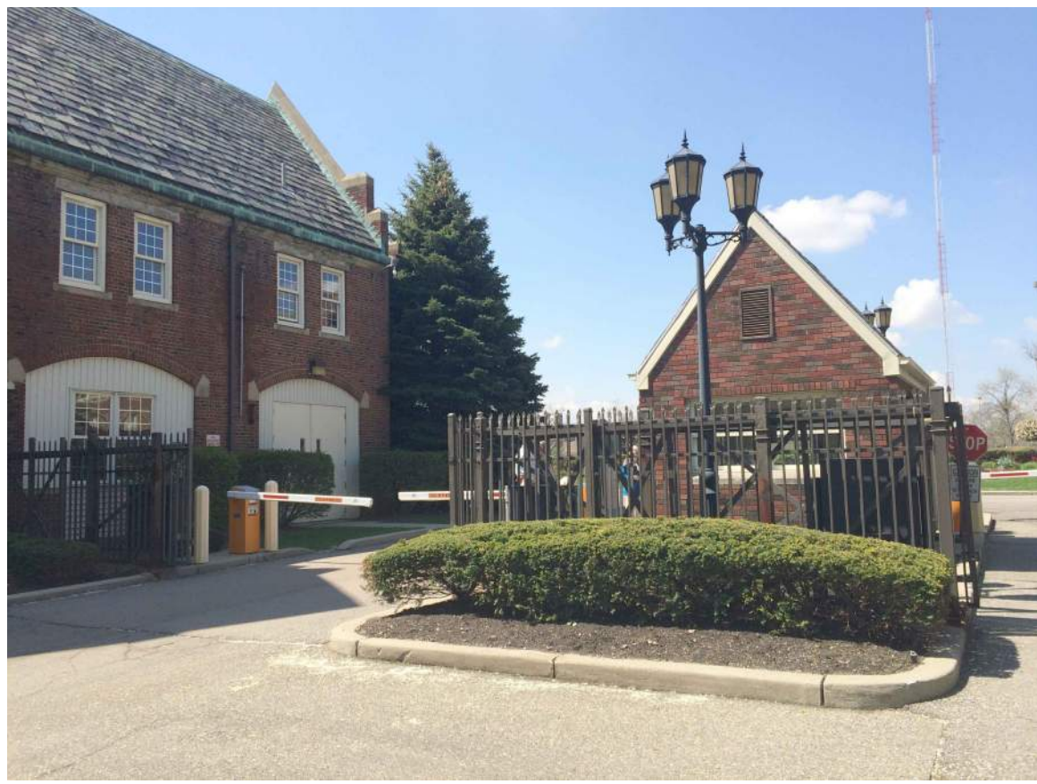
REFERENCE PHOTO 01 EXISTING GATE HOUSE
