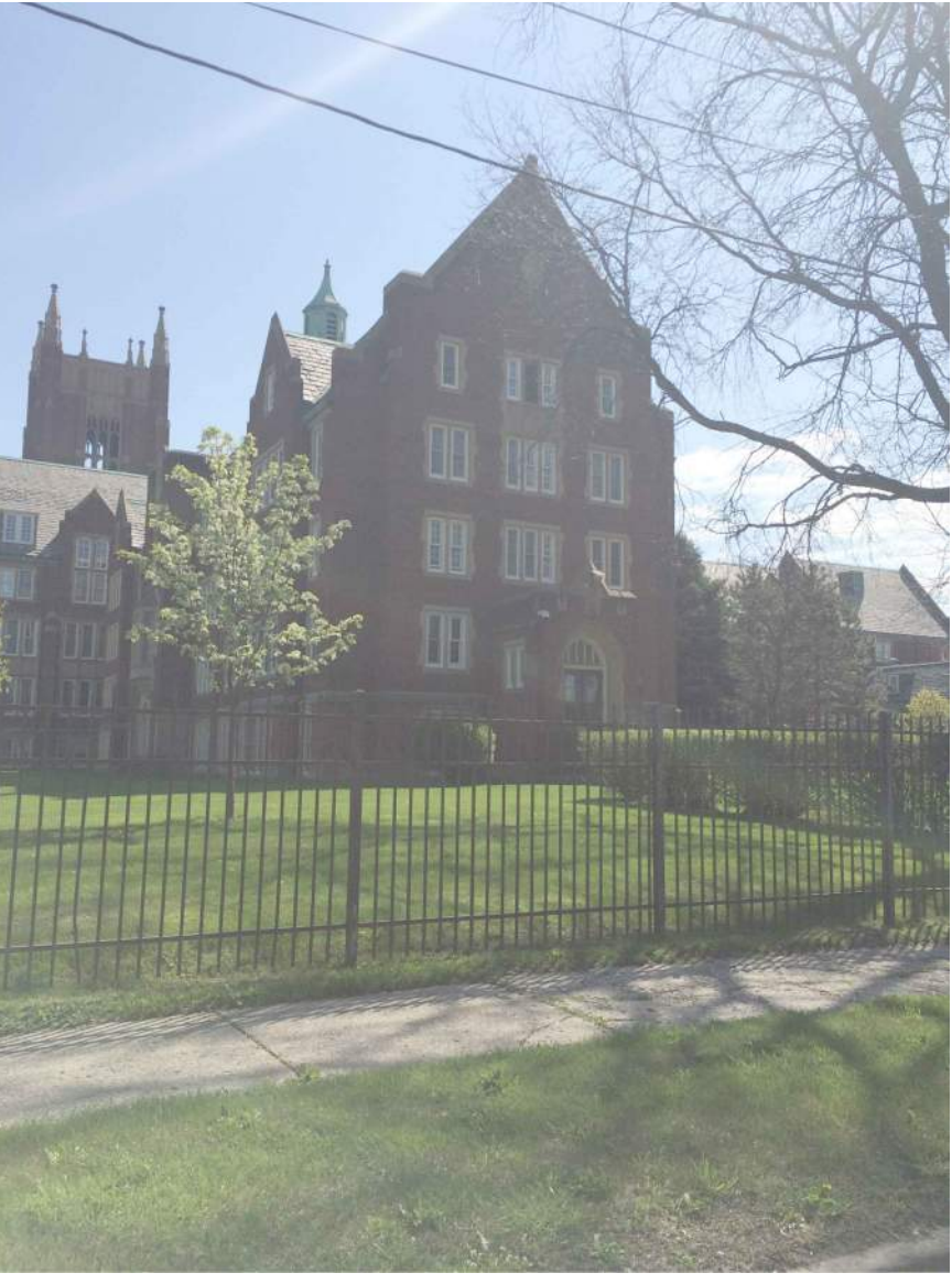
REFERENCE PHOTO 05 EXISTING BUILDING ADJACENT TO NEW GUARD HOUSE
