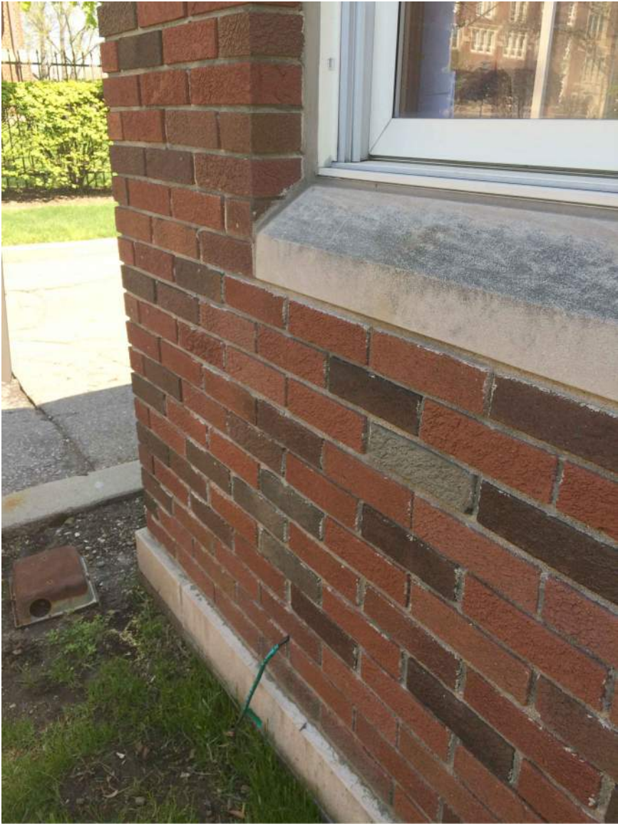
REFERENCE PHOTO 03 EXISTING GATE HOUSE
