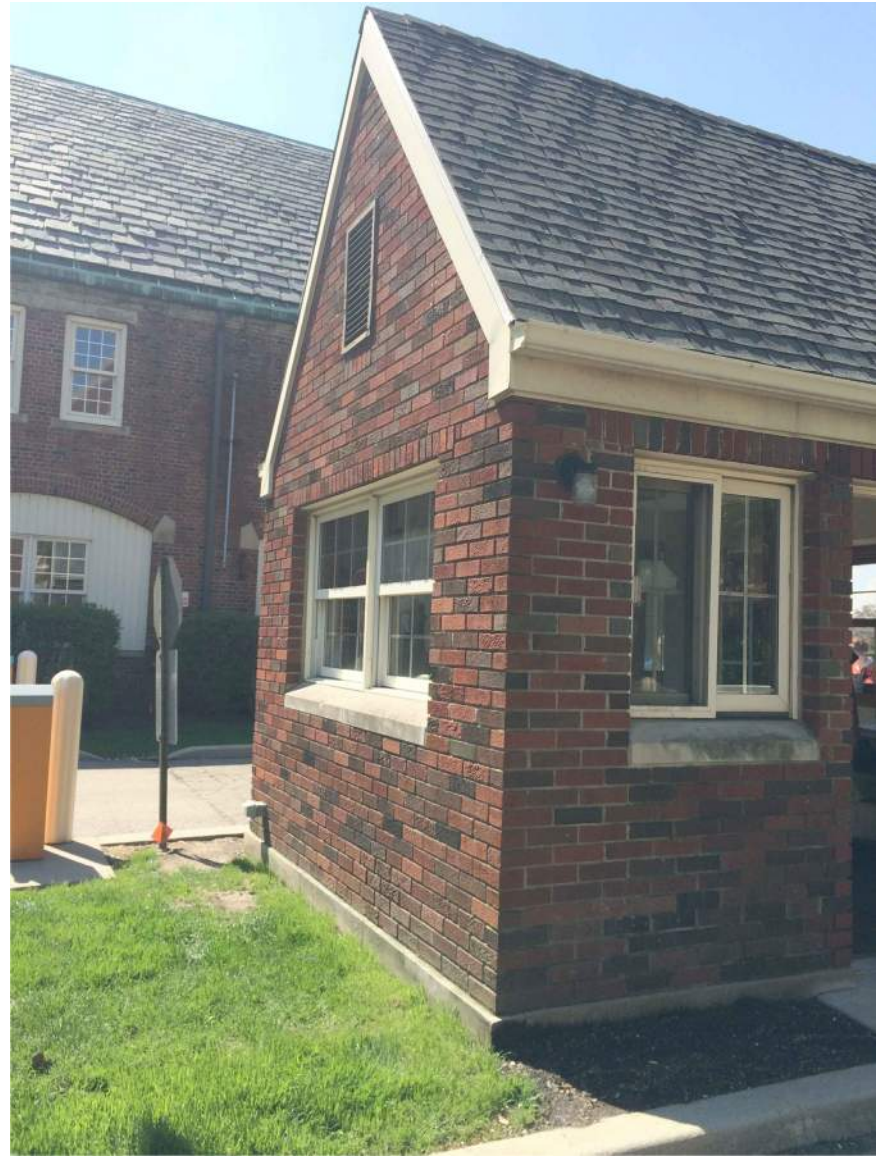
REFERENCE PHOTO 04 EXISTING GATE HOUSE
