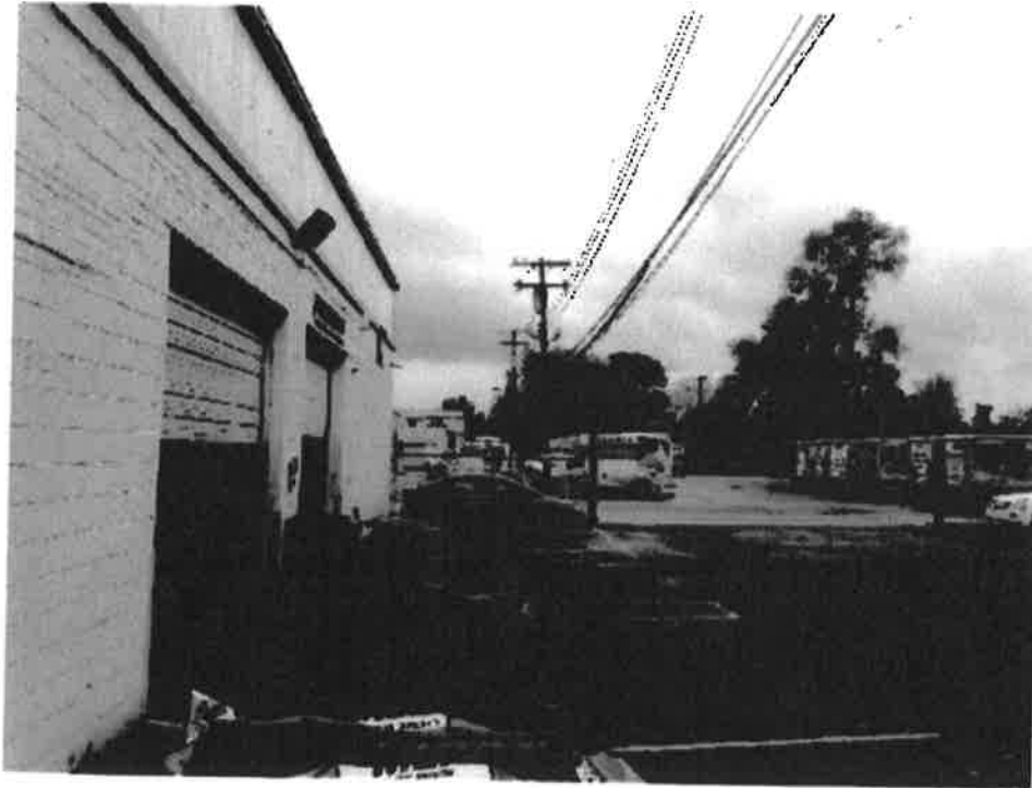
The lane is approximately 2 feet off the building and inside the utility poles. A portion of the lane is now grass.
