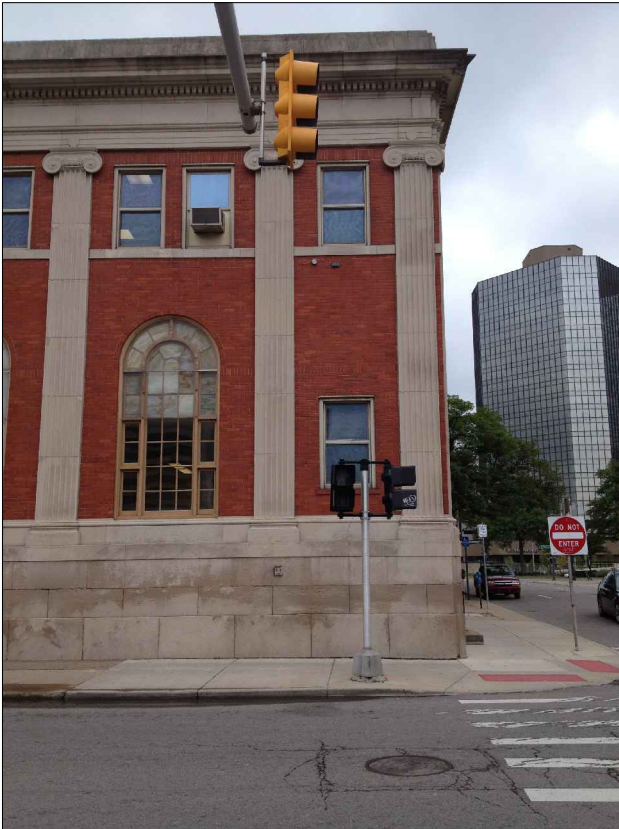
VIEW SOUTH TOWARDS INTERSECTION OF LARNED & ST. ANTOINE
