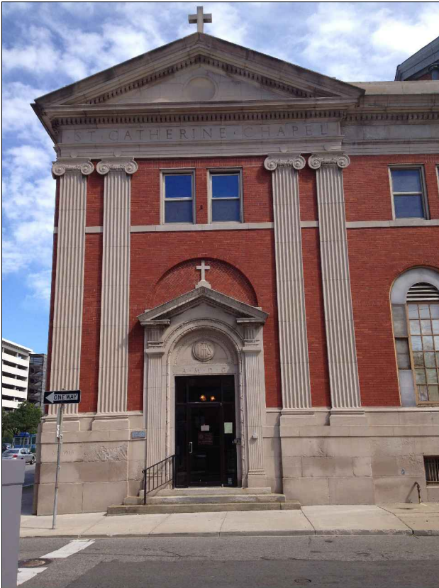
VIEW EAST TOWARDS EXISTING ST. ANTOINE ENTRY
