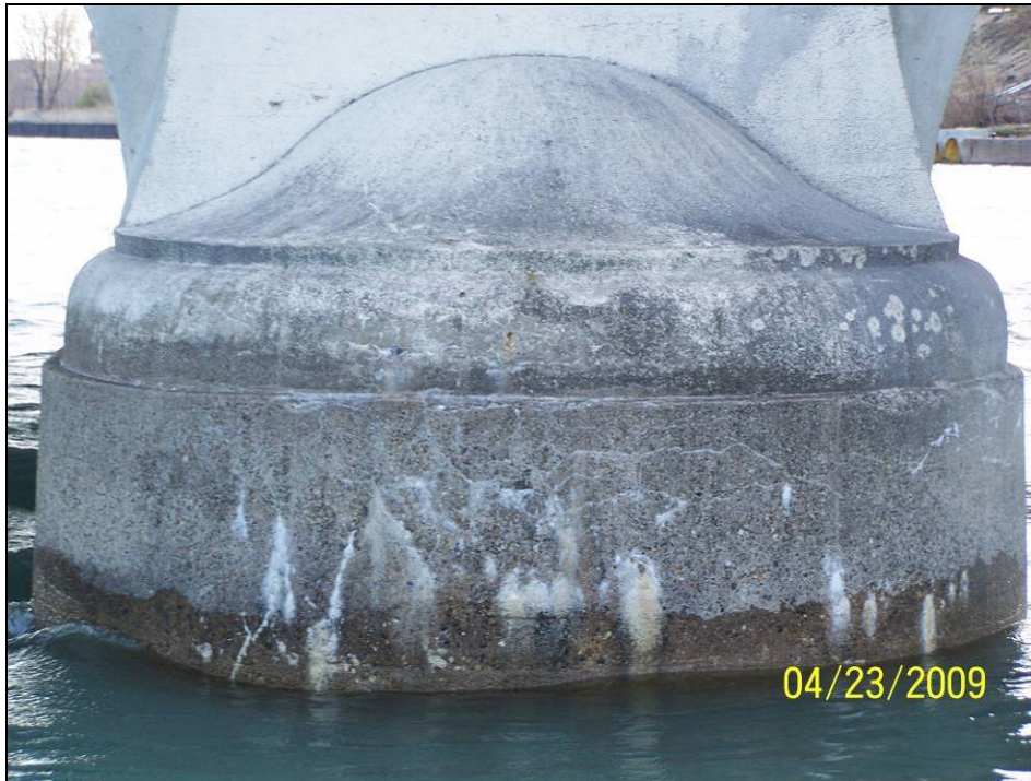
Photograph 13. View of Pier 2 Upstream Nose.
