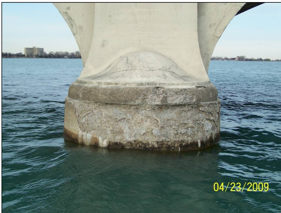
Photograph 42. View of Pier 9 Downstream Nose.
