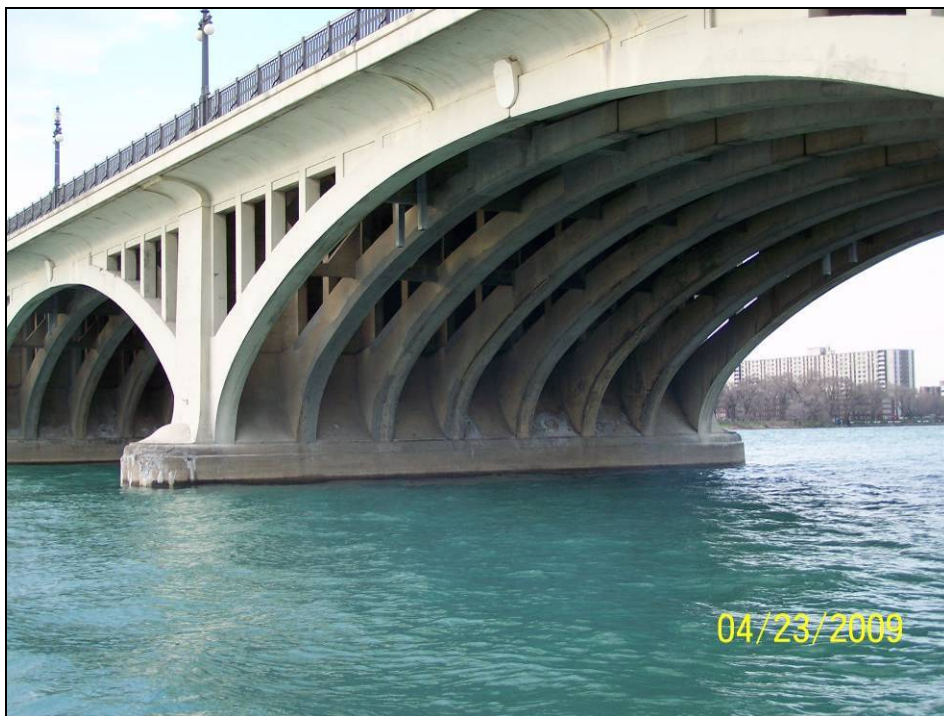
Photograph 36. View of Pier 8 South Face.
