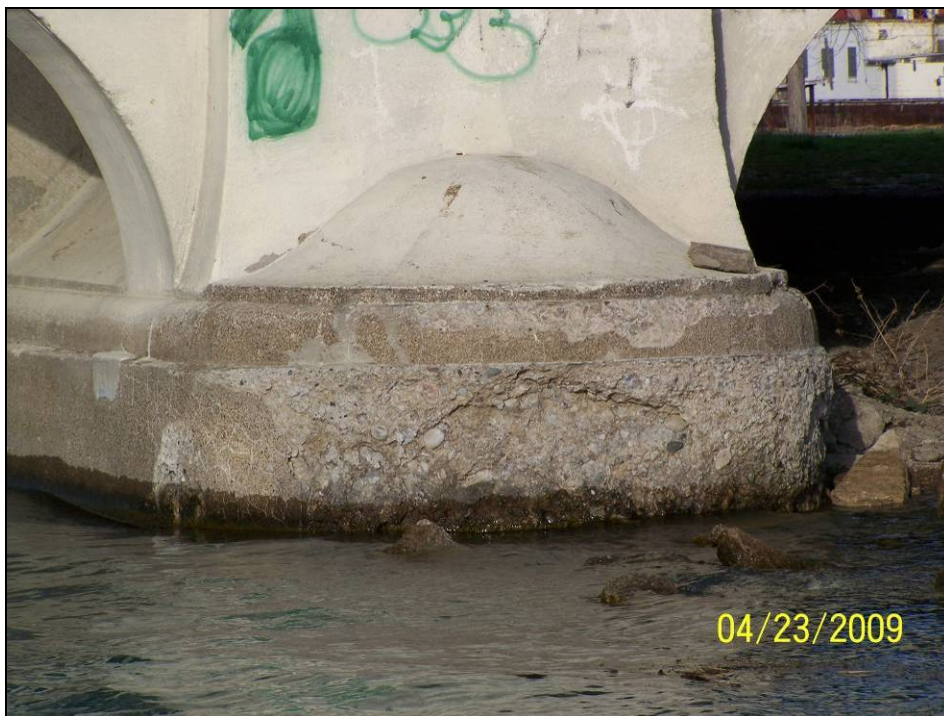
Photograph 78. View of Pier 18 Downstream Nose.
