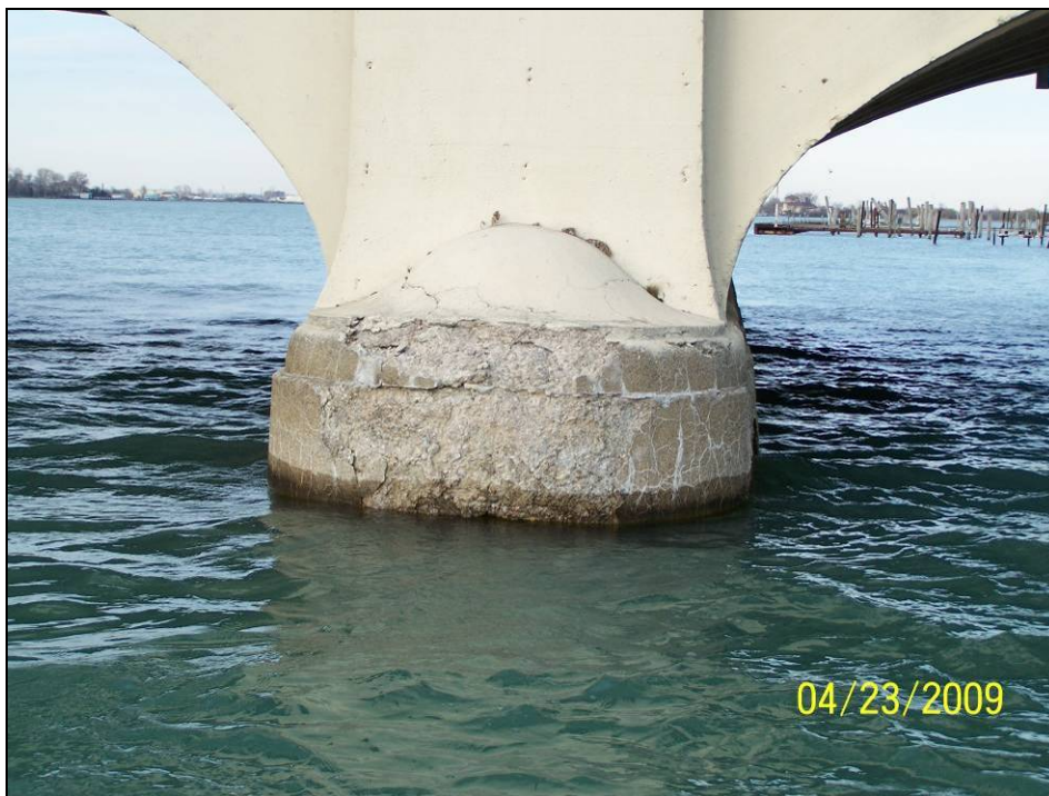
Photograph 74. View of Pier 17 Downstream Nose.
