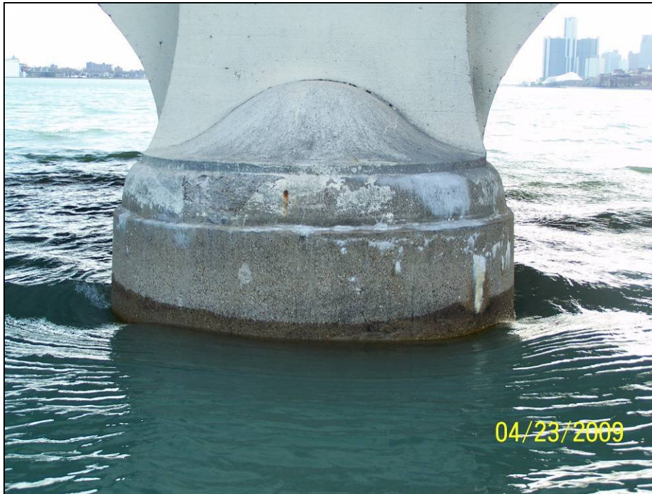
Photograph 65. View of Pier 15 Upstream Nose.
