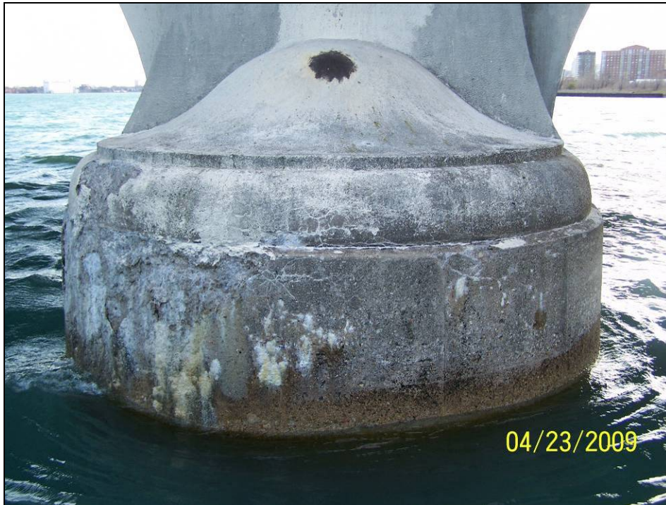
Photograph 21. View of Pier 4 Upstream Nose.
