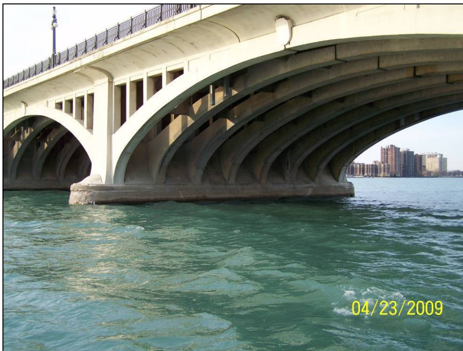
Photograph 52. View of Pier 12 South Face.
