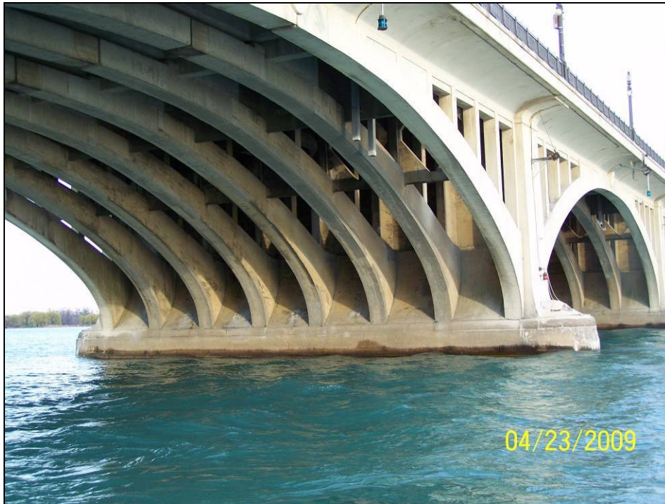
Photograph 23. View of Pier 5 North Face.
