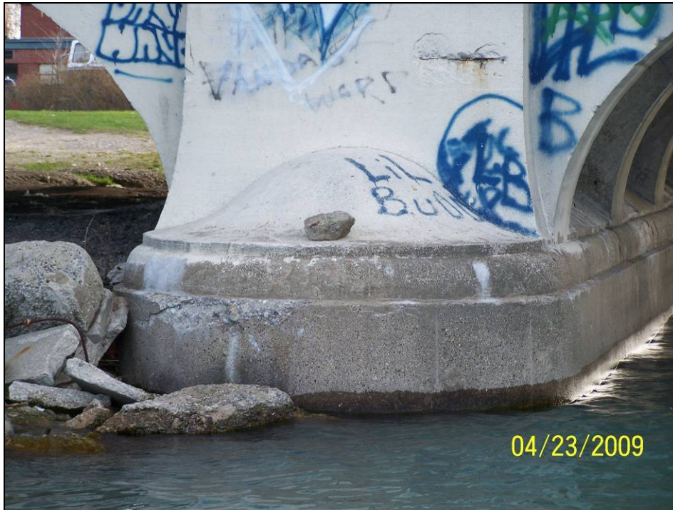
Photograph 77. View of Pier 18 Upstream Nose.
