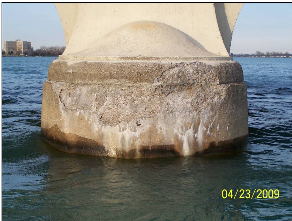
Photograph 30. View of Pier 6 Downstream Nose.
