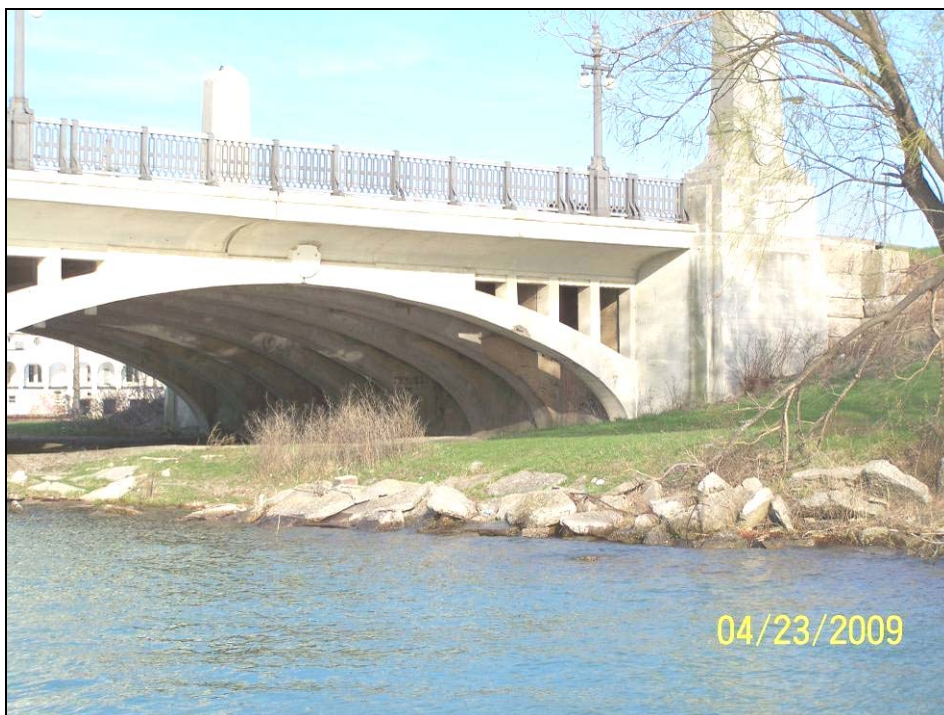
Photograph 80: View of South Abutment, North Face and West Face.
