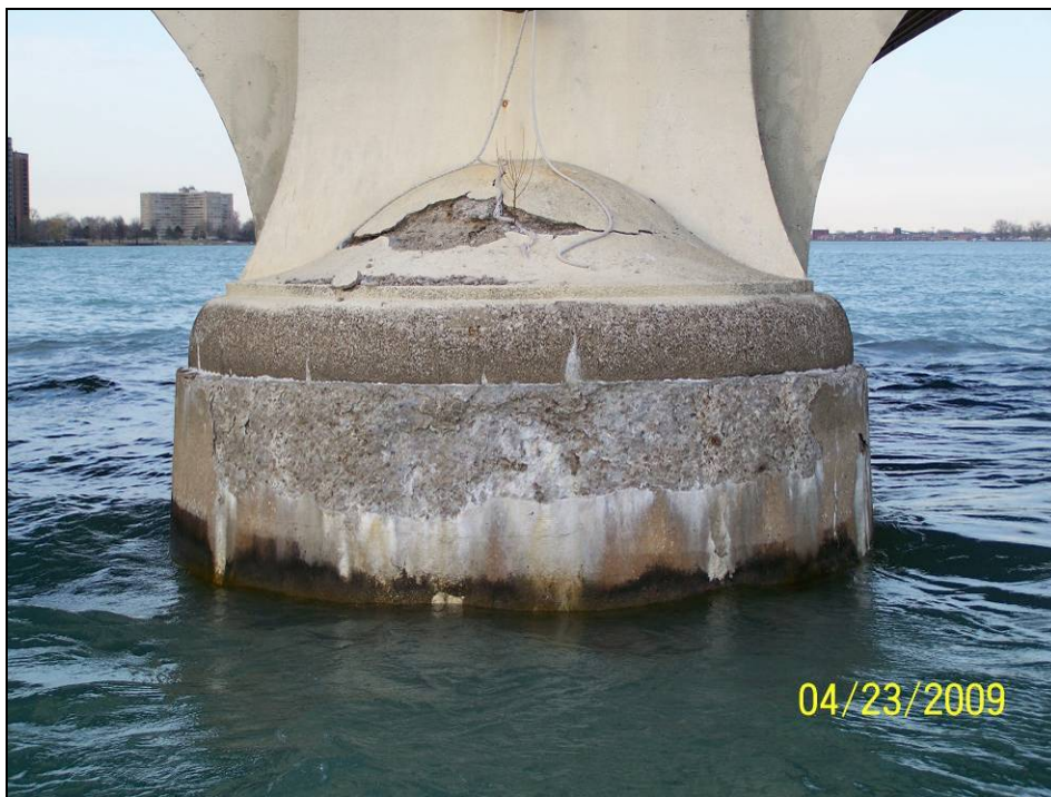
Photograph 26. View of Pier 5 Downstream Nose.
