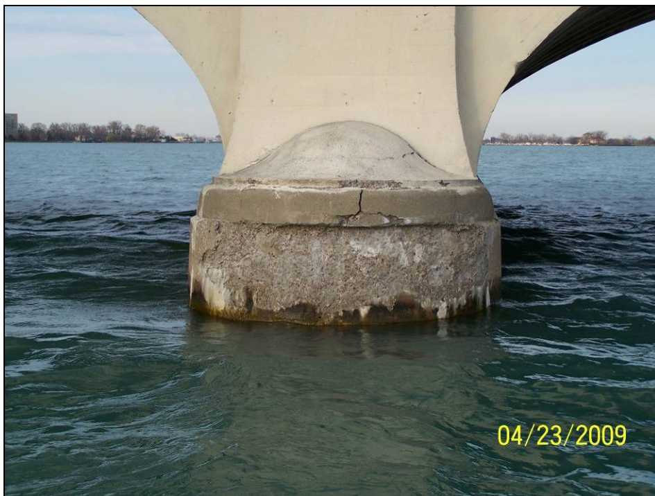
Photograph 54. View of Pier 12 Downstream Nose.
