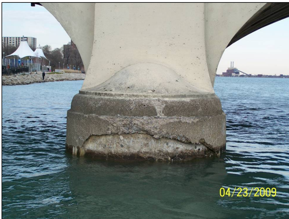
Photograph 10. View of Pier 1 Downstream Nose.
