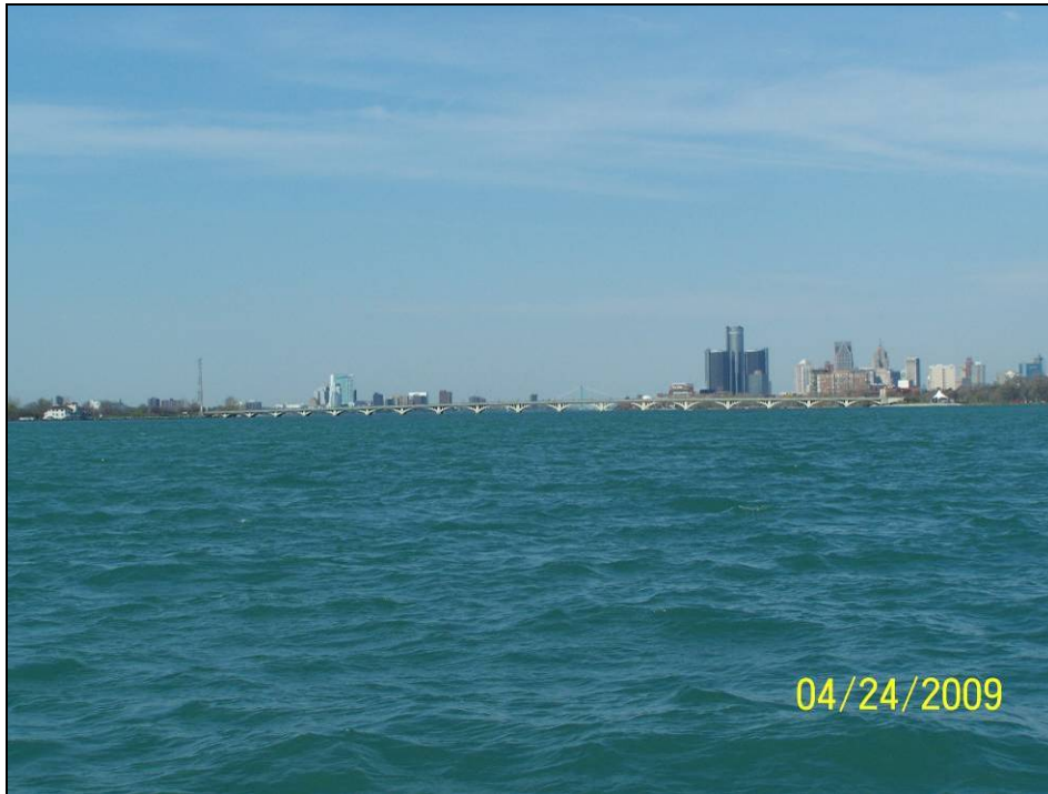
Photograph 1. Overall View of the Upstream Fascia.
