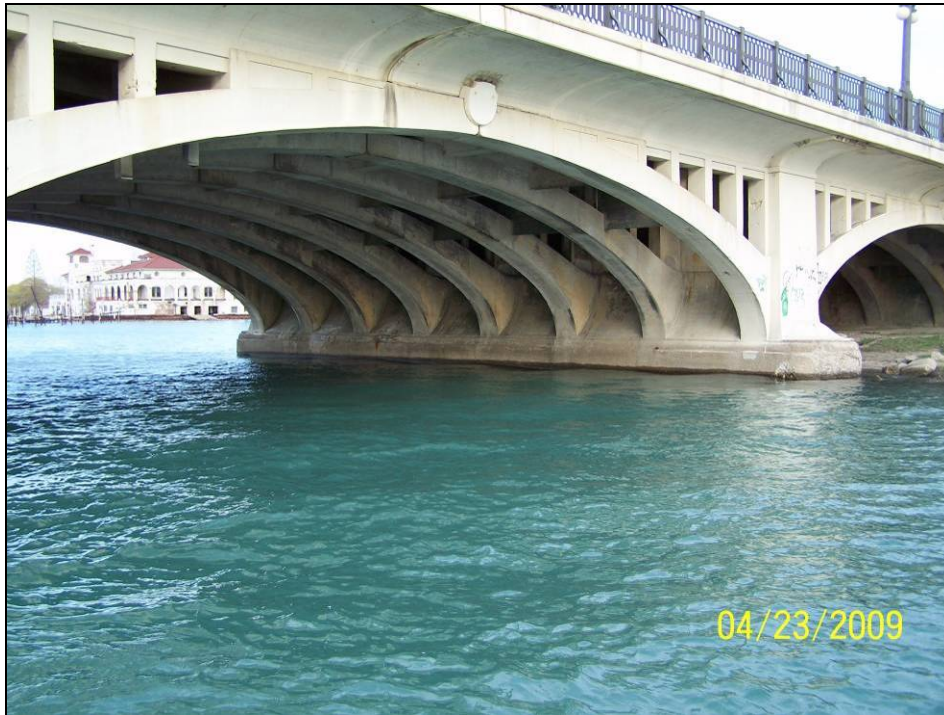
Photograph 75. View of Pier 18 North Face.
