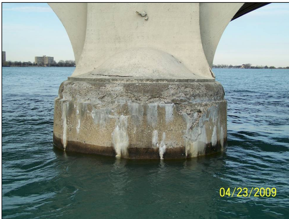
Photograph 38. View of Pier 8 Downstream Nose.
