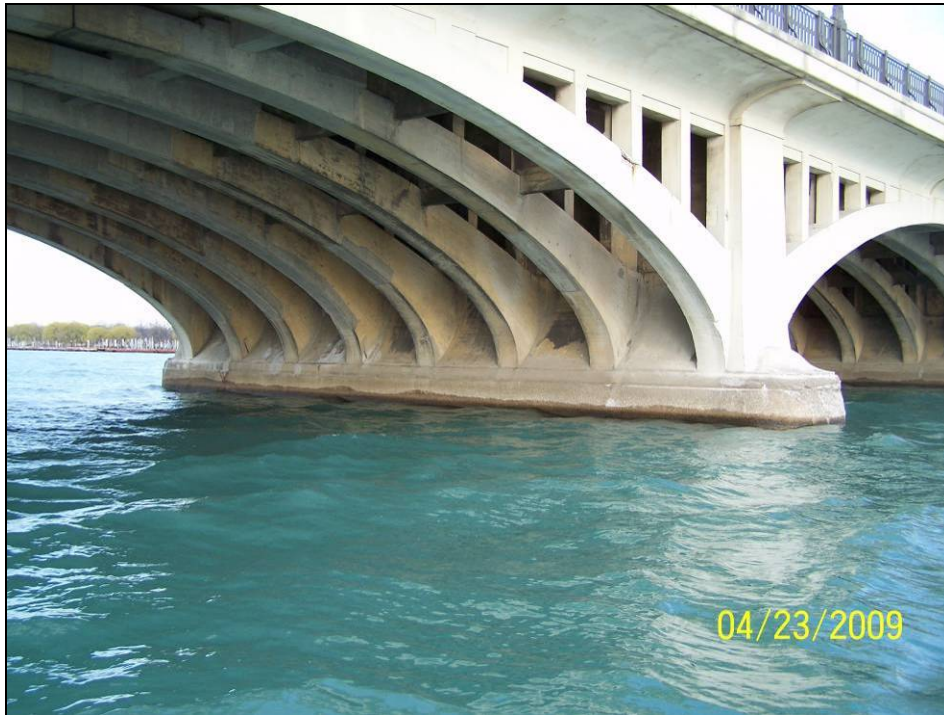
Photograph 59. View of Pier 14 North Face.
