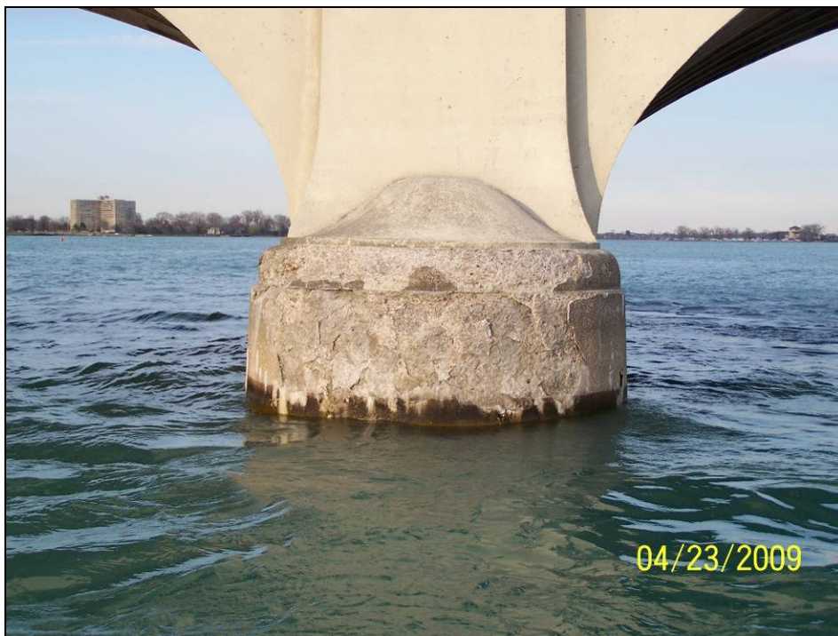
Photograph 34. View of Pier 7 Downstream Nose.
