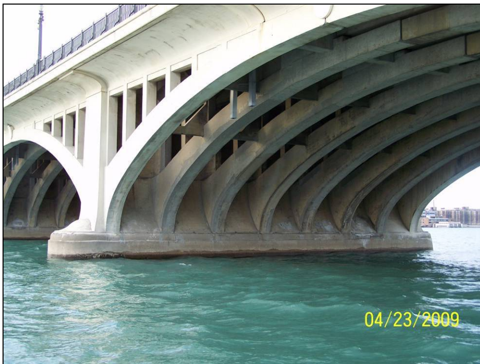
Photograph 48. View of Pier 11 South Face.
