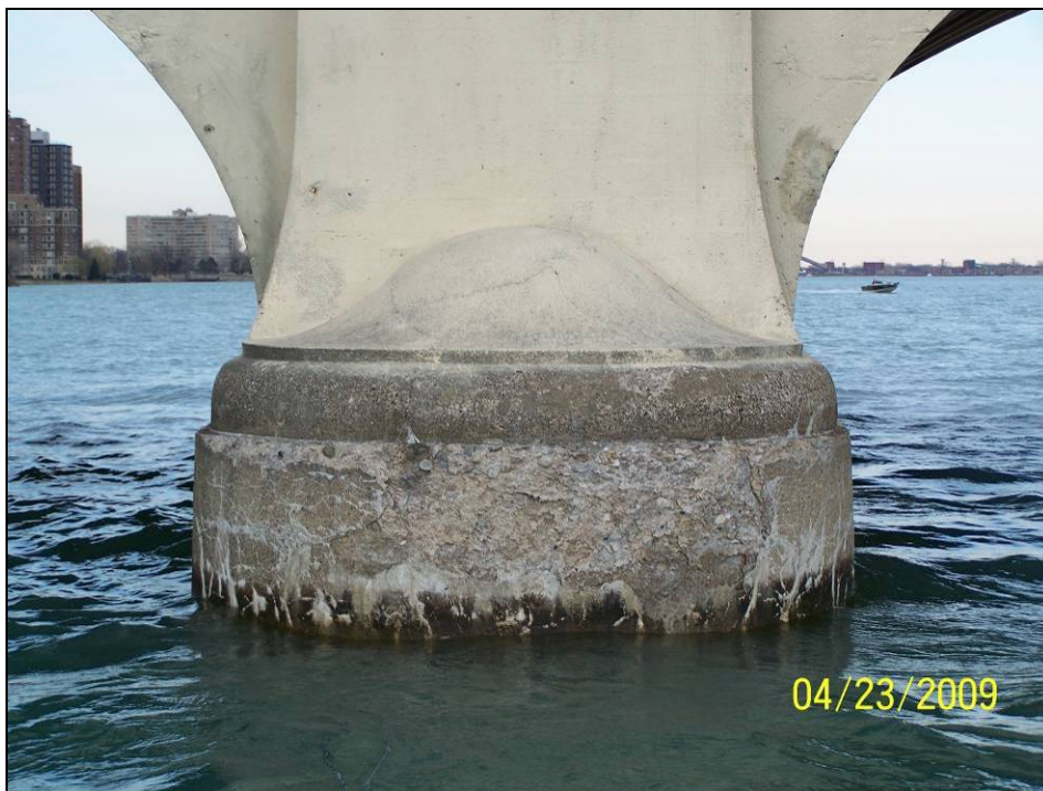
Photograph 14. View of Pier 2 Downstream Nose.
