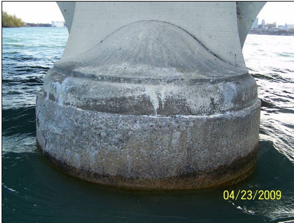
Photograph 61. View of Pier 14 Upstream Nose.
