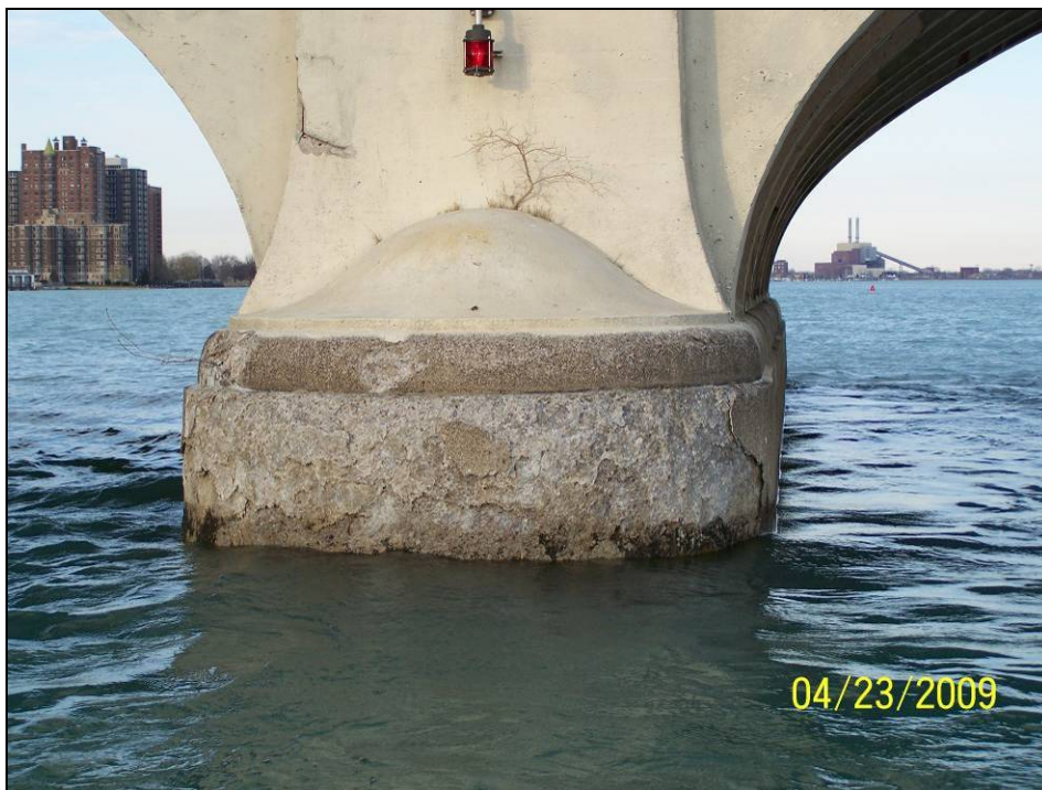
Photograph 22. View of Pier 4 Downstream Nose.
