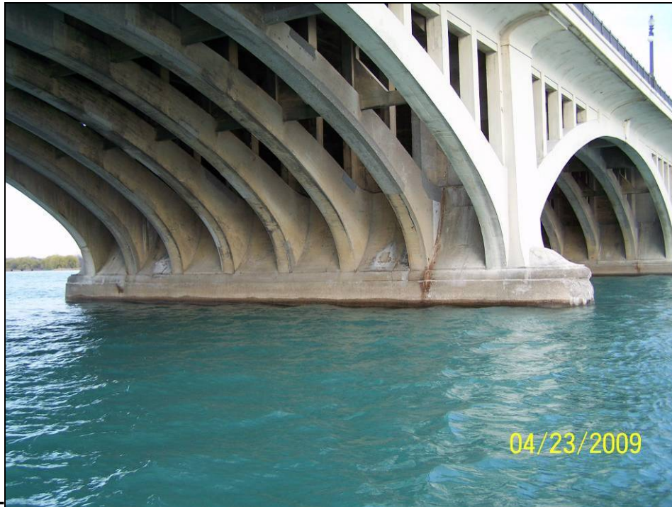
Photograph 39. View of Pier 9 North Face.
