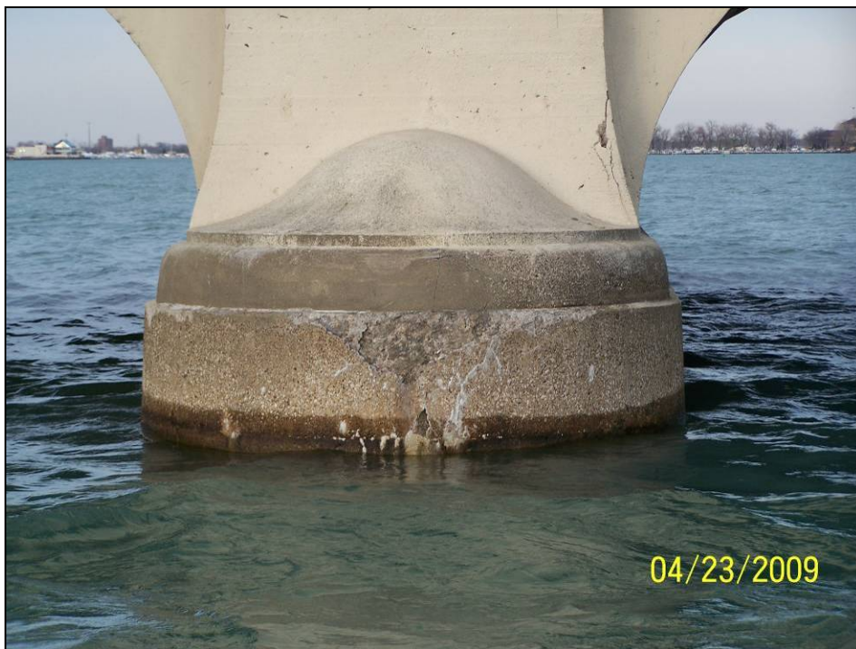
Photograph 58. View of Pier 13 Downstream Nose.
