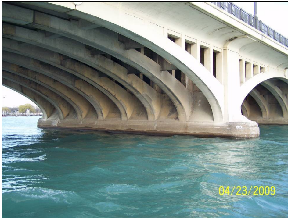
Photograph 63. View of Pier 15 North Face.
