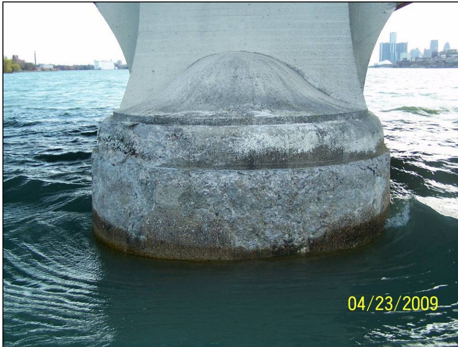
Photograph 57. View of Pier 13 Upstream Nose.
