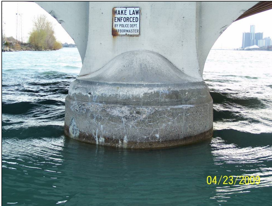
Photograph 69. View of Pier 16 Upstream Nose.
