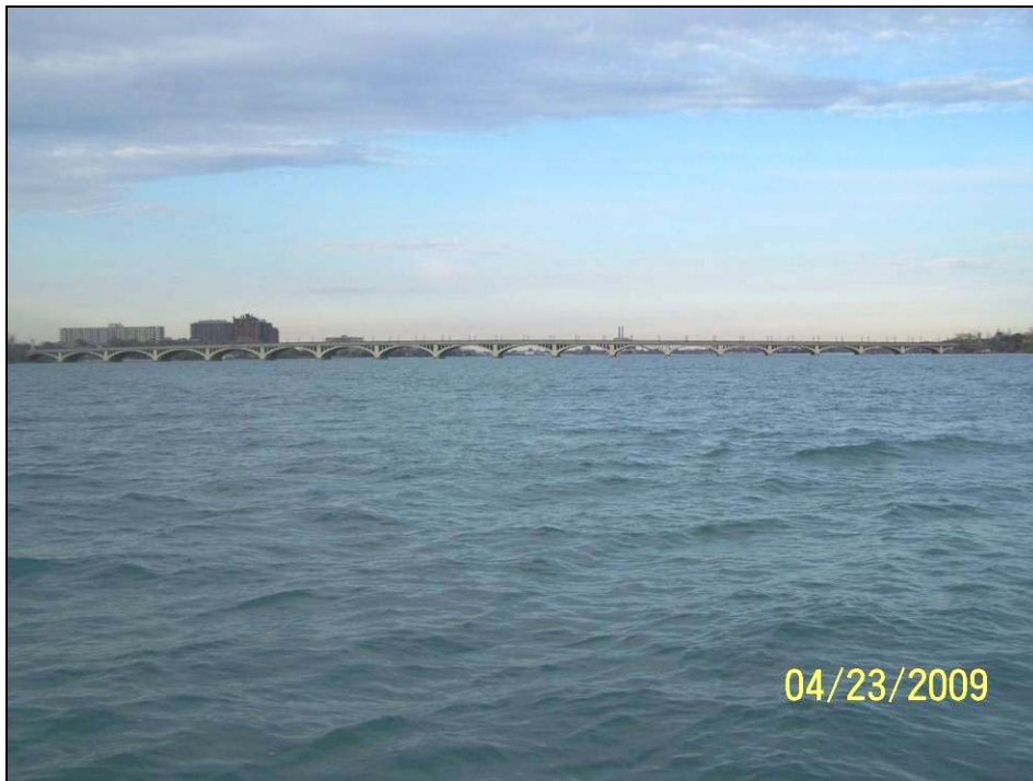
Photograph 2. Overall View of the Downstream Fascia.
