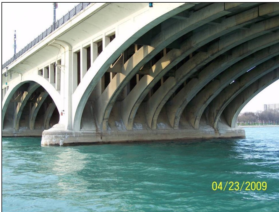
Photograph 24. View of Pier 5 South Face.
