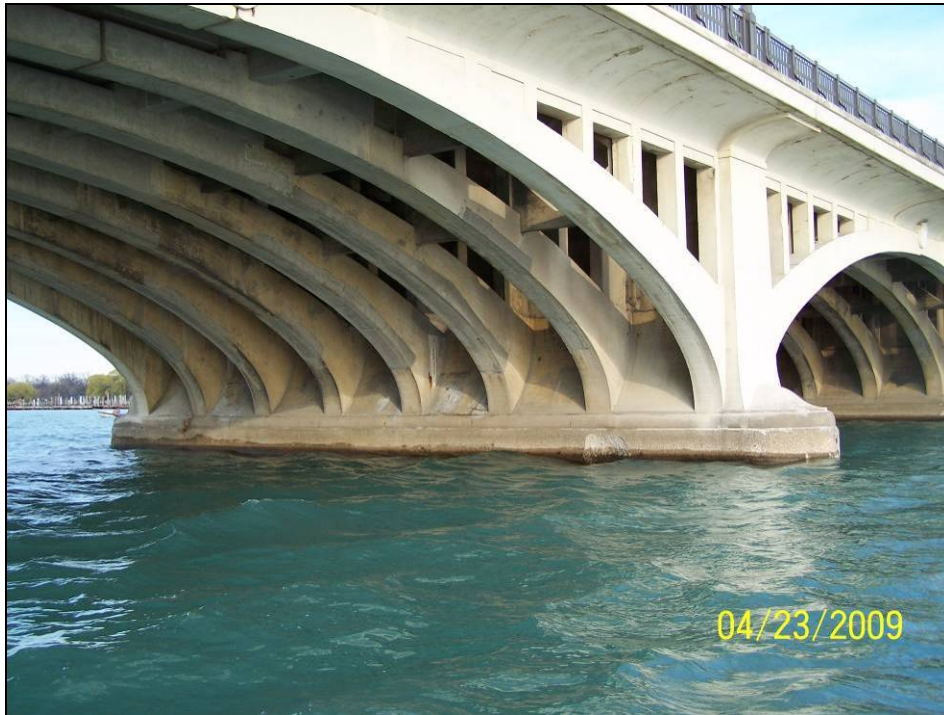
Photograph 55. View of Pier 13 North Face.
