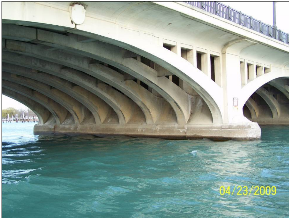
Photograph 67. View of Pier 16 North Face.
