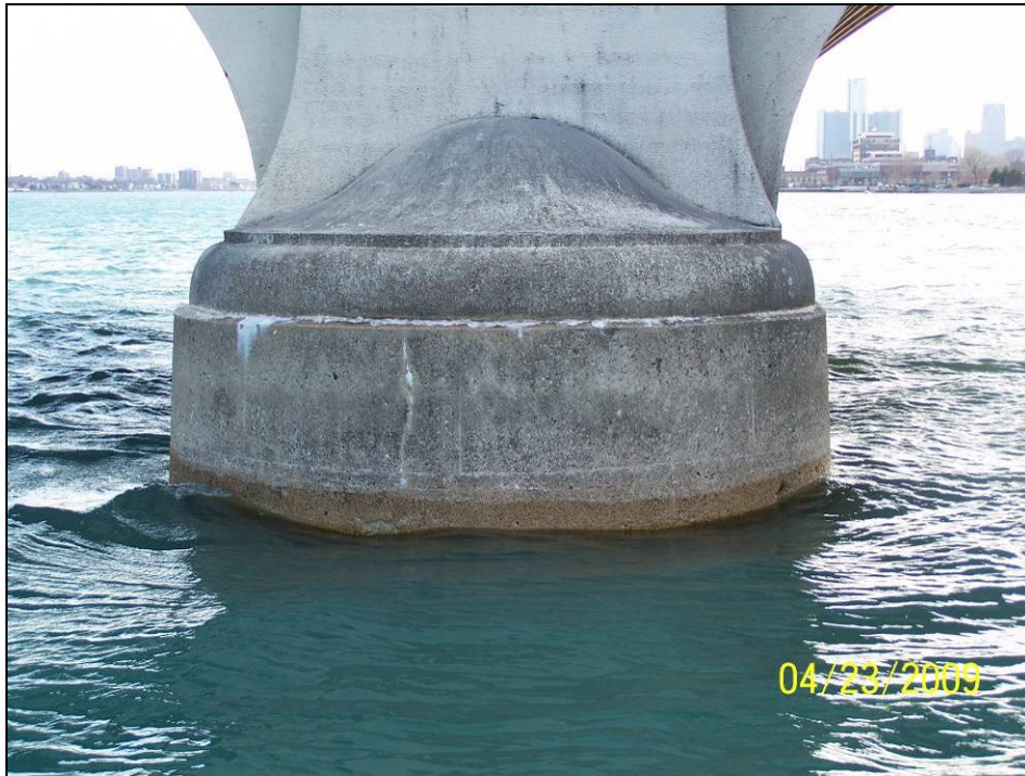
Photograph 37. View of Pier 8 Upstream Nose.
