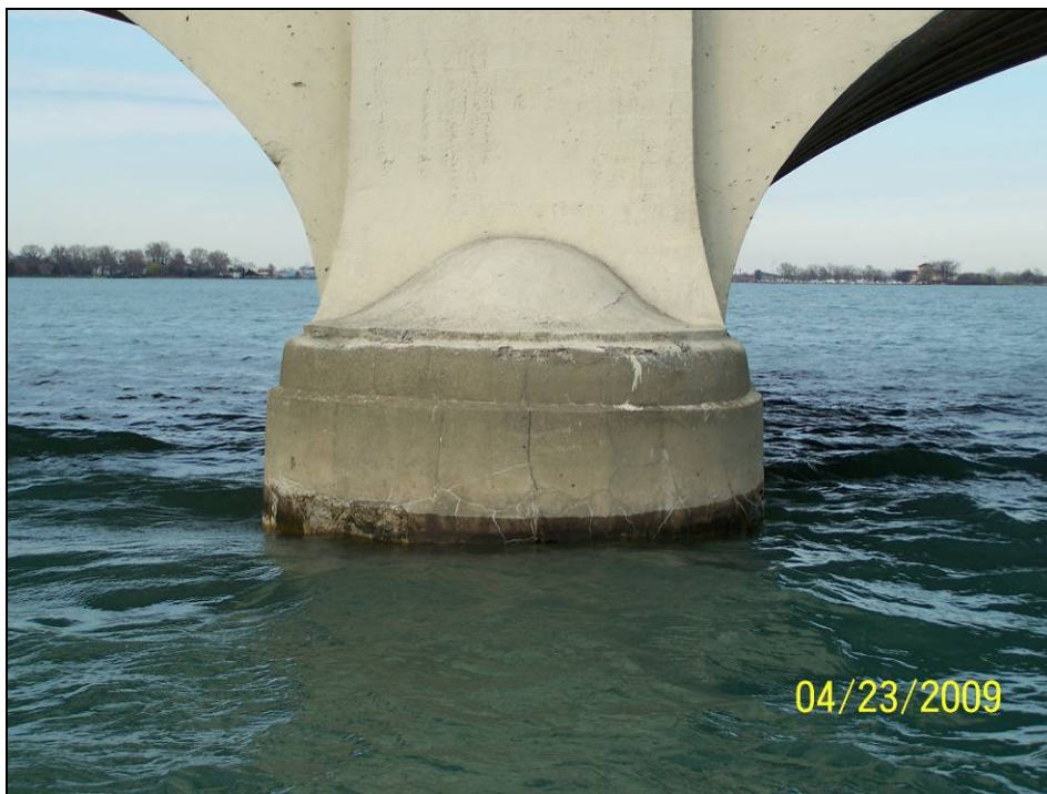
Photograph 50. View of Pier 11 Downstream Nose.
