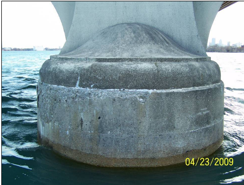
Photograph 33. View of Pier 7 Upstream Nose.
