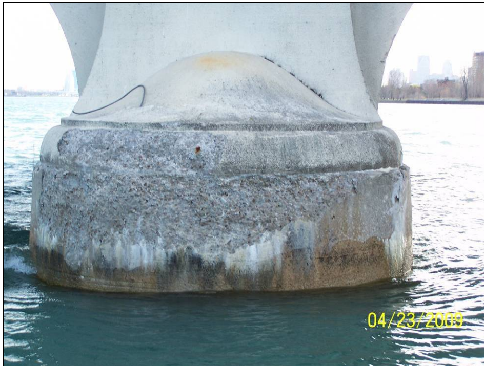
Photograph 25. View of Pier 5 Upstream Nose.
