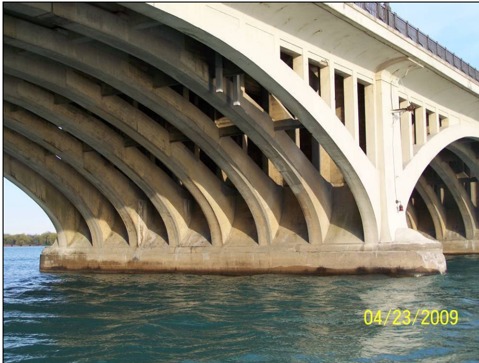
Photograph 27. View of Pier 6 North Face.
