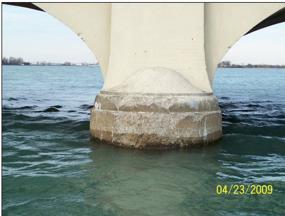
Photograph 66. View of Pier 15 Downstream Nose.
