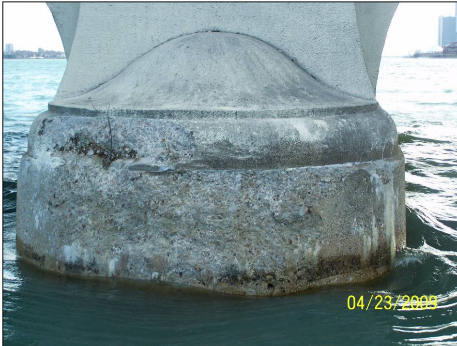
Photograph 49. View of Pier 11 Upstream Nose.
