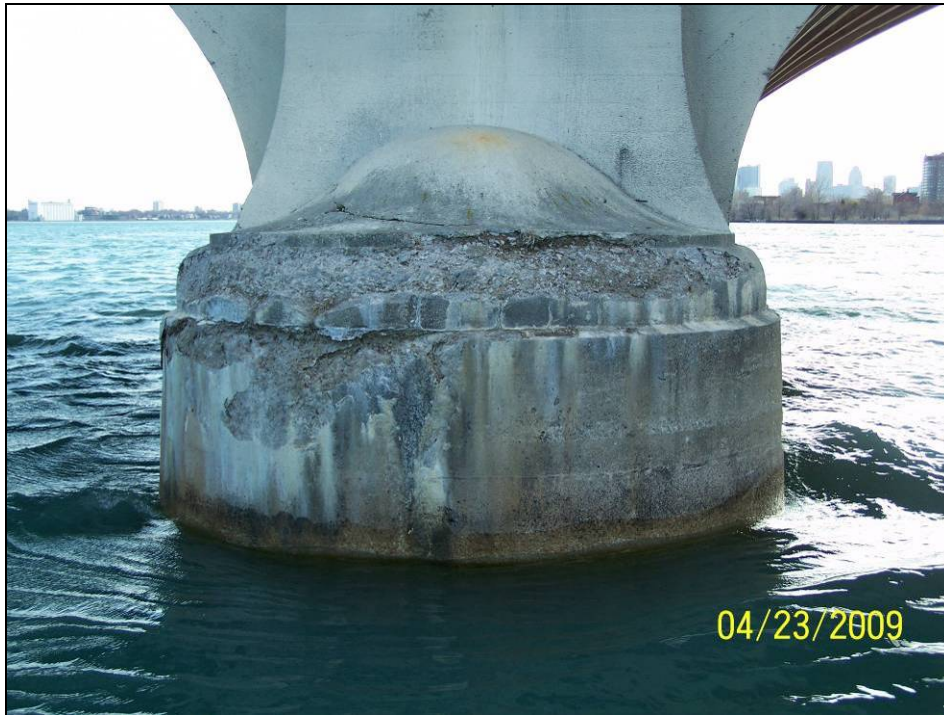
Photograph 29. View of Pier 6 Upstream Nose.
