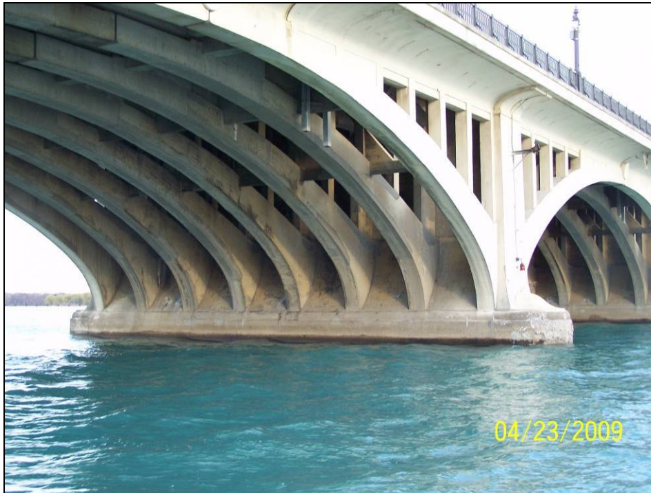
Photograph 19. View of Pier 4 North Face.
