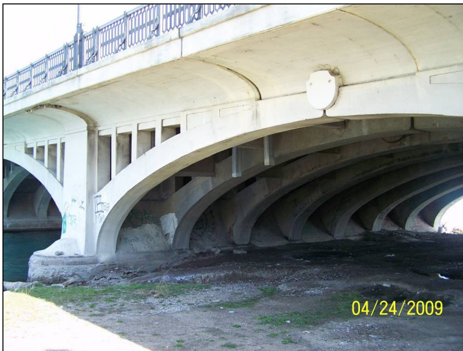
Photograph 76. View of Pier 18 South Face.
