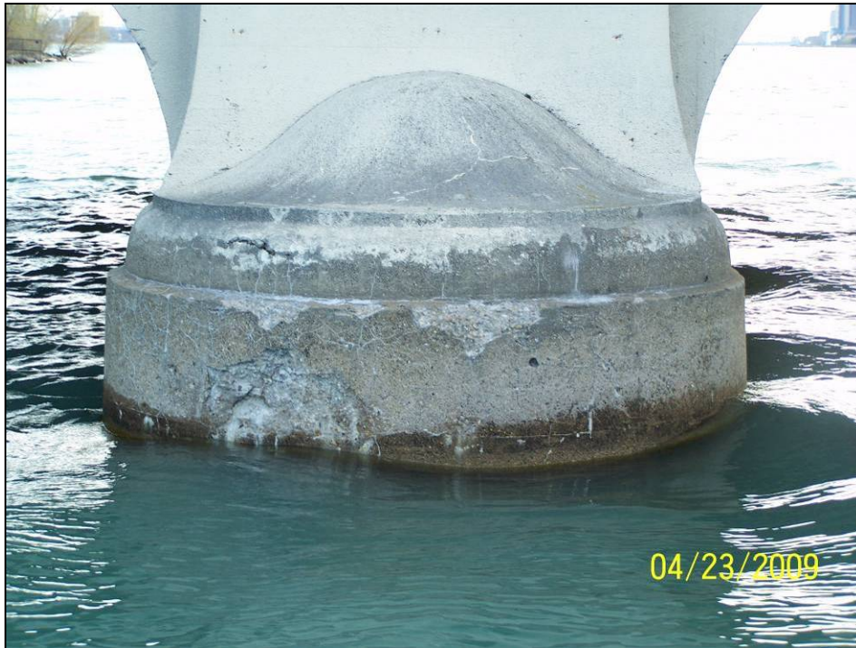
Photograph 73. View of Pier 17 Upstream Nose.
