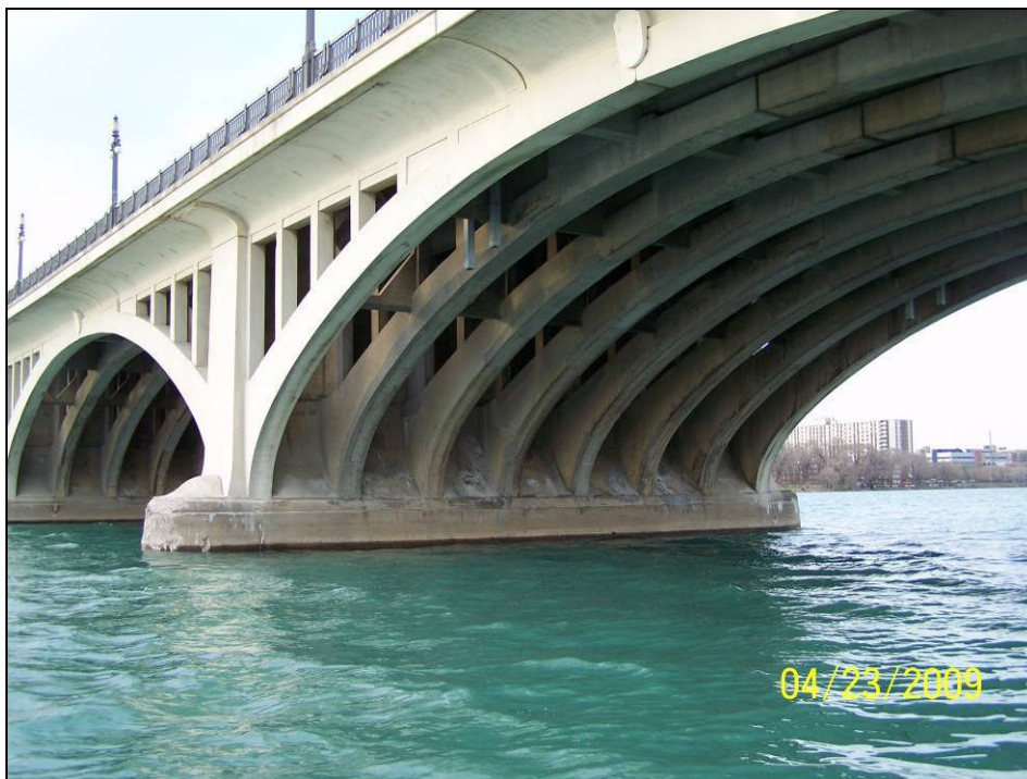
Photograph 32. View of Pier 7 South Face.
