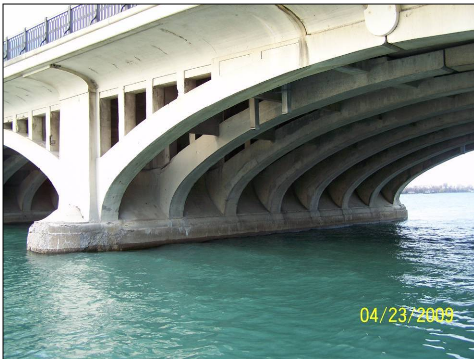
Photograph 72. View of Pier 17 South Face.
