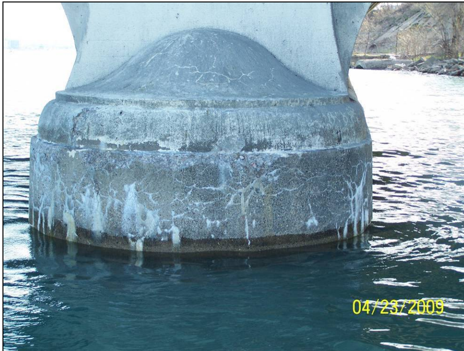
Photograph 9. View of Pier 1 Upstream Nose.
