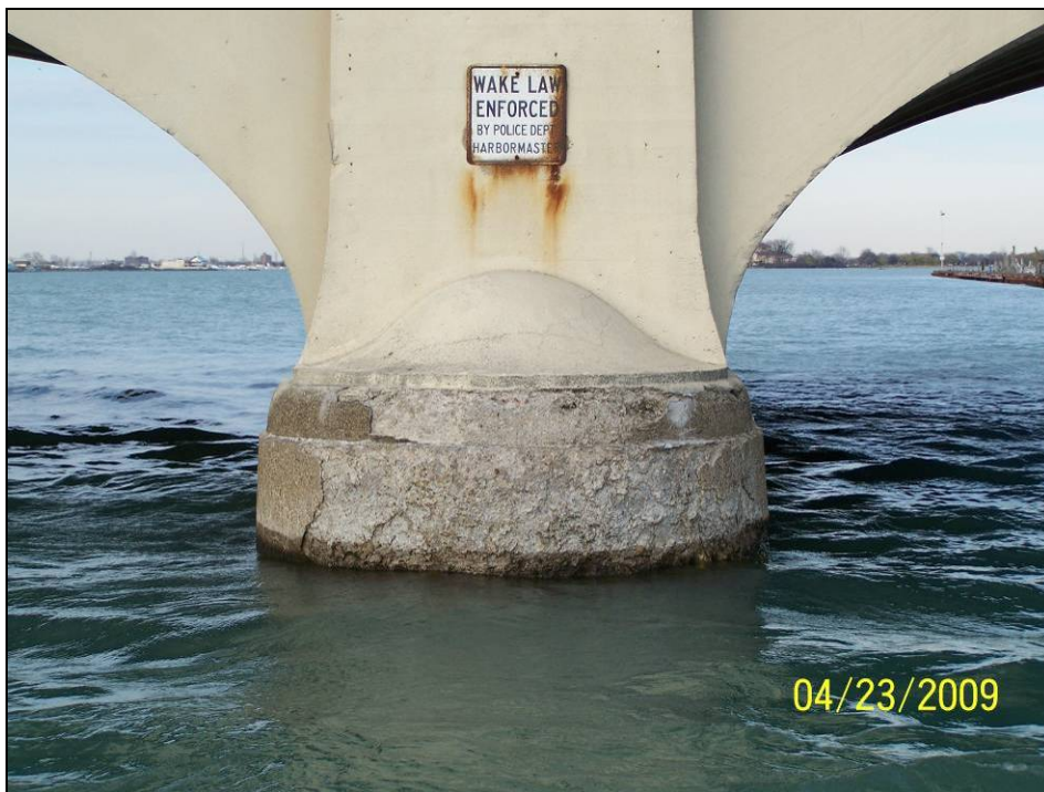
Photograph 70. View of Pier 16 Downstream Nose.
