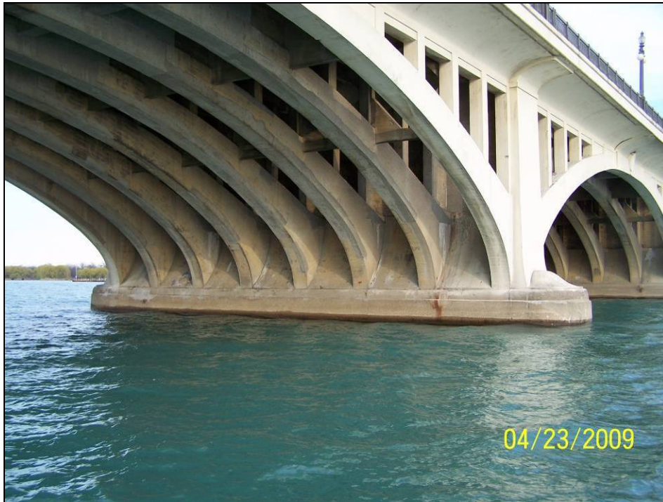
Photograph 43. View of Pier 10 North Face.
