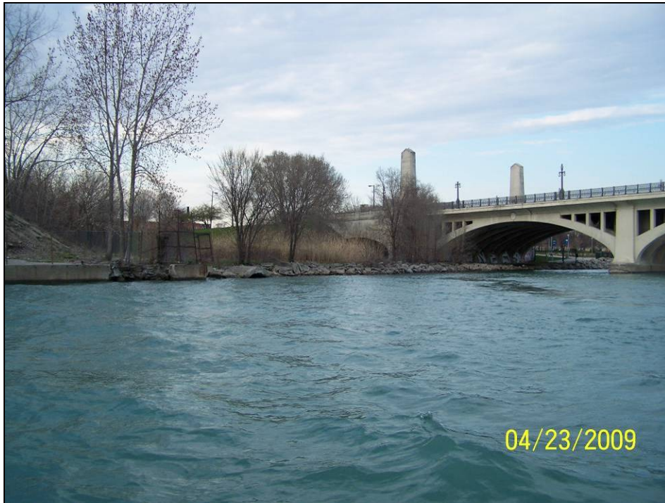
Photograph 81: View of the Northwest Embankment.
