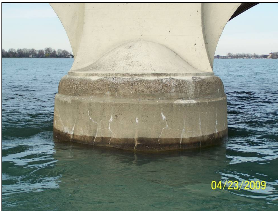
Photograph 46. View of Pier 10 Downstream Nose.
