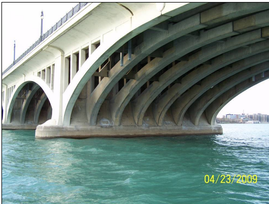
Photograph 44. View of Pier 10 South Face.
