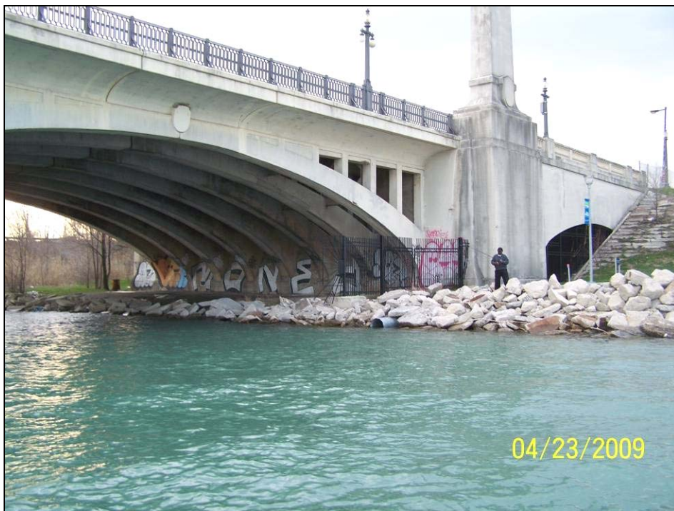
Photograph 6. View of Abutment A, South Face and East Face.
