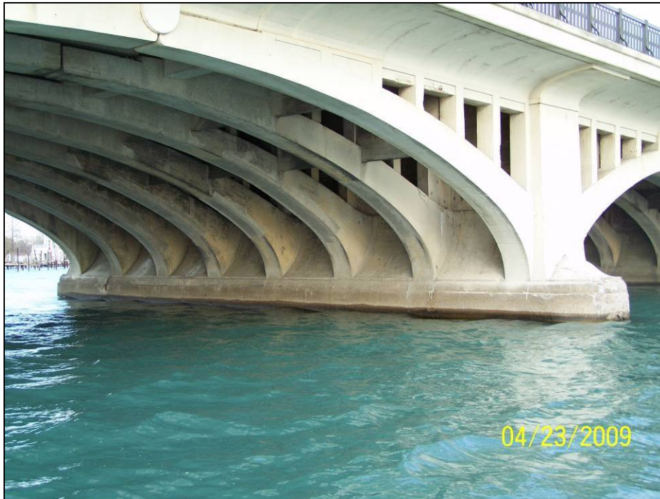
Photograph 71. View of Pier 17 North Face.
