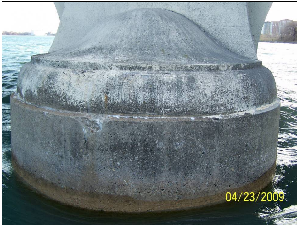
Photograph 17. View of Pier 3 Upstream Nose.
