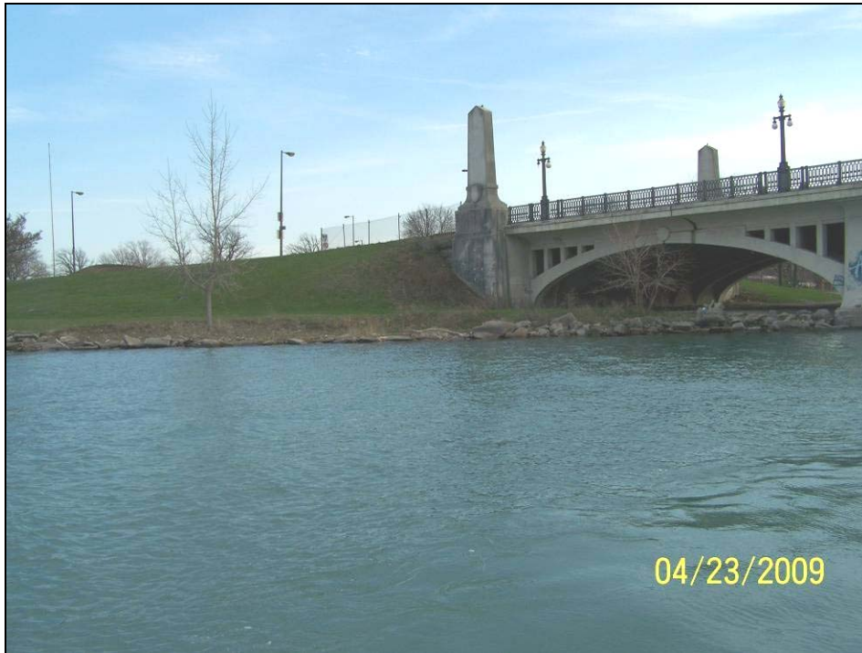
Photograph 83: View of the Southeast Embankment.
