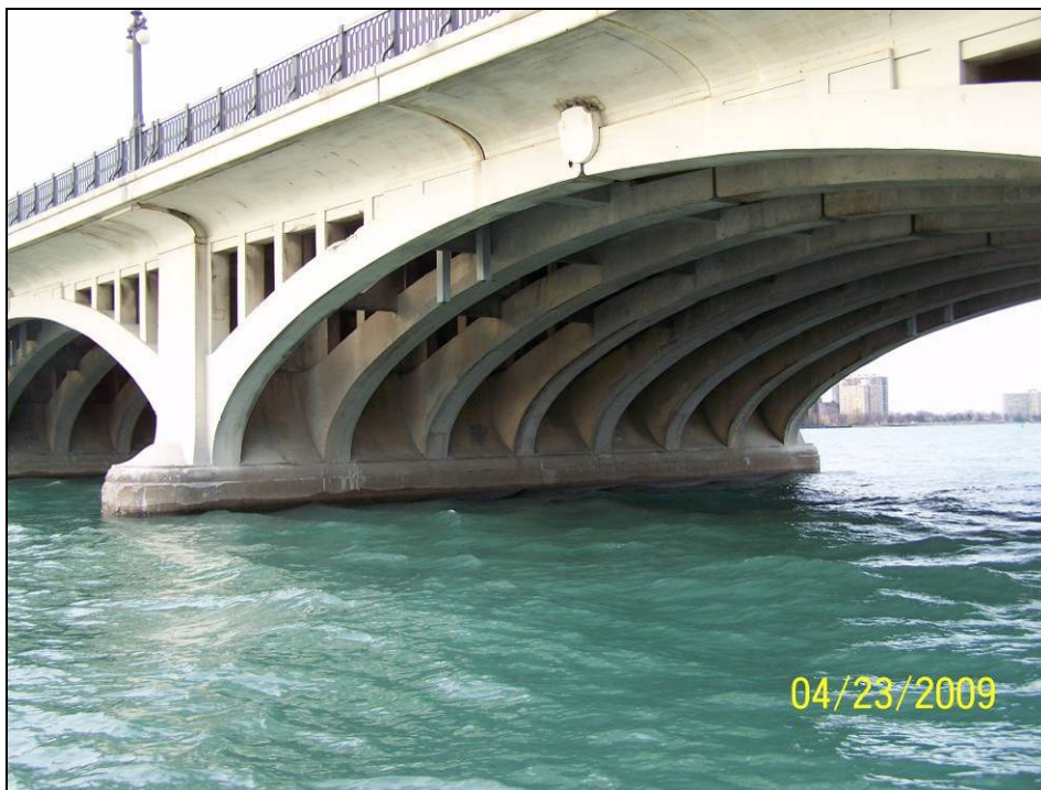
Photograph 64. View of Pier 15 South Face.
