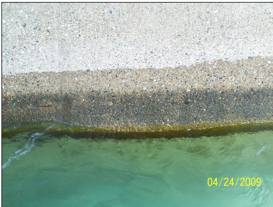
Photograph 88: View of Typical Concrete Condition Near the Waterline.
