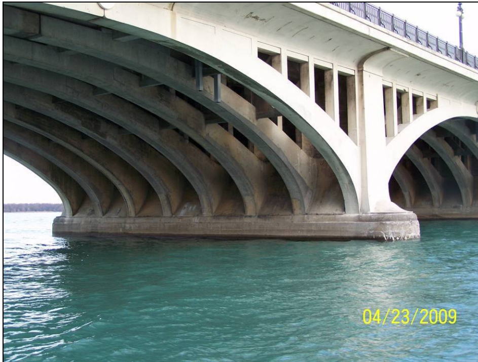
Photograph 11. View of Pier 2 North Face.
