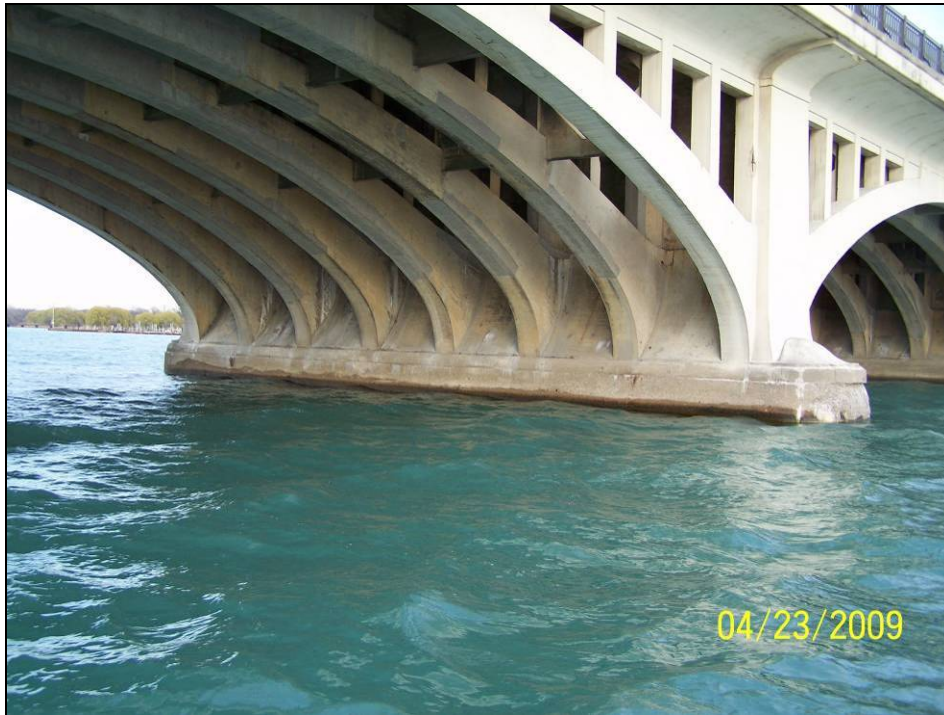
Photograph 51. View of Pier 12 North Face.
