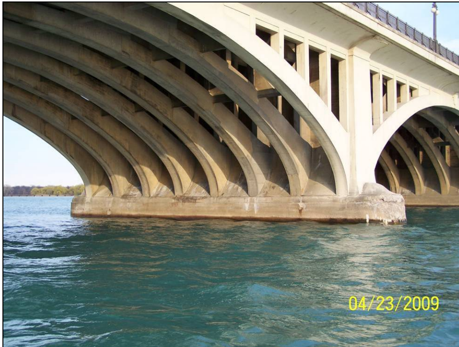
Photograph 31. View of Pier 7 North Face.
