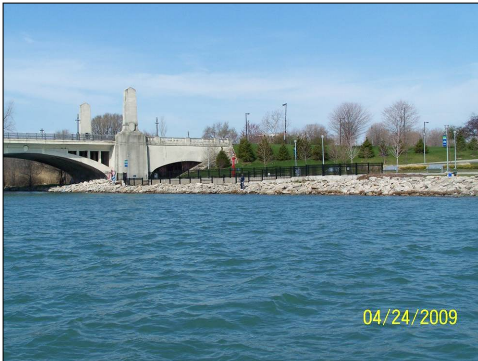
Photograph 82: View of the Northeast Embankment.
