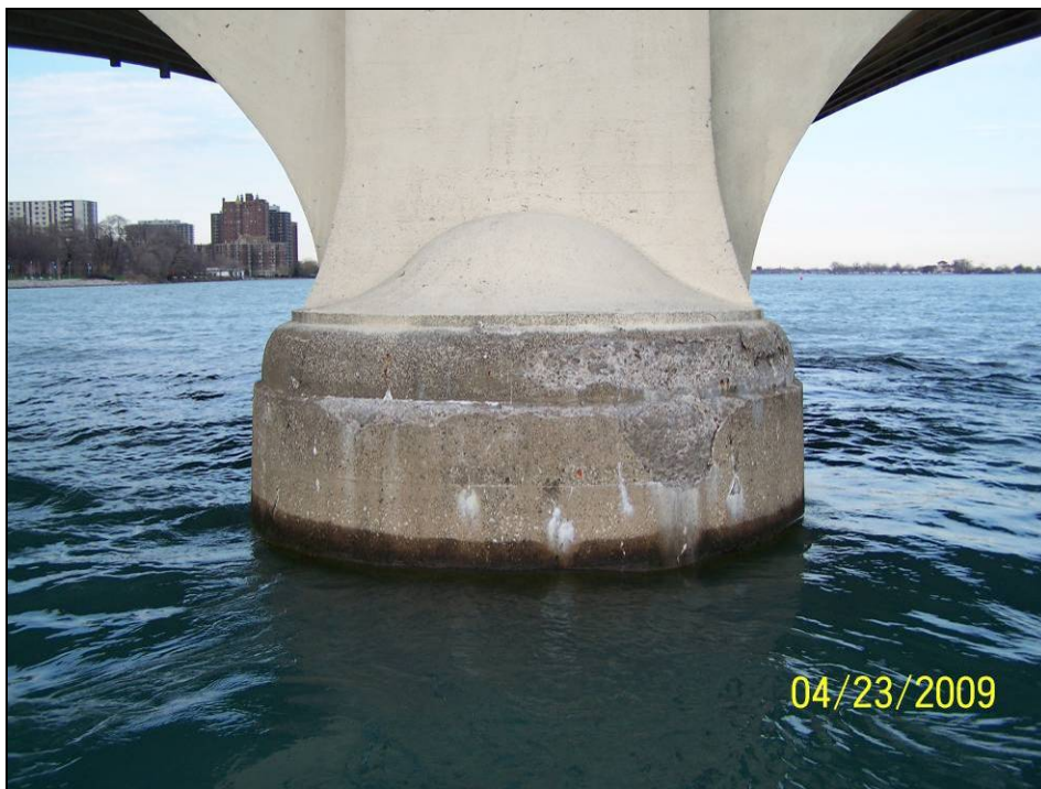
Photograph 18. View of Pier 3 Downstream Nose.
