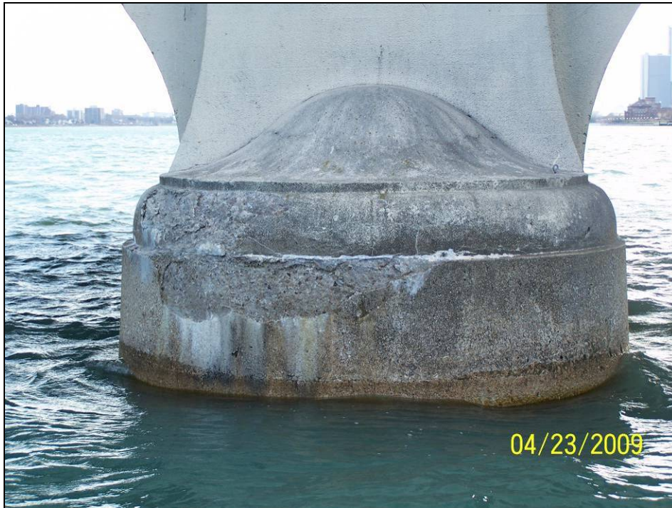
Photograph 45. View of Pier 10 Upstream Nose.
