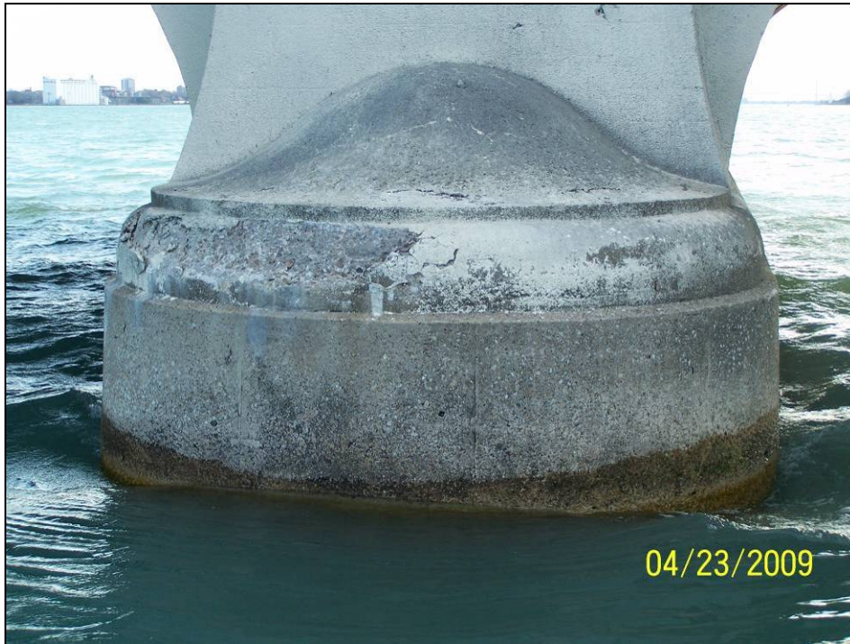
Photograph 53. View of Pier 12 Upstream Nose.
