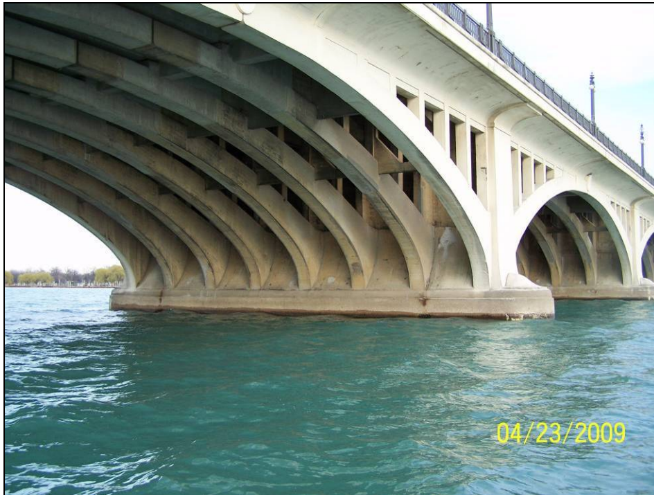
Photograph 47. View of Pier 11 North Face.
