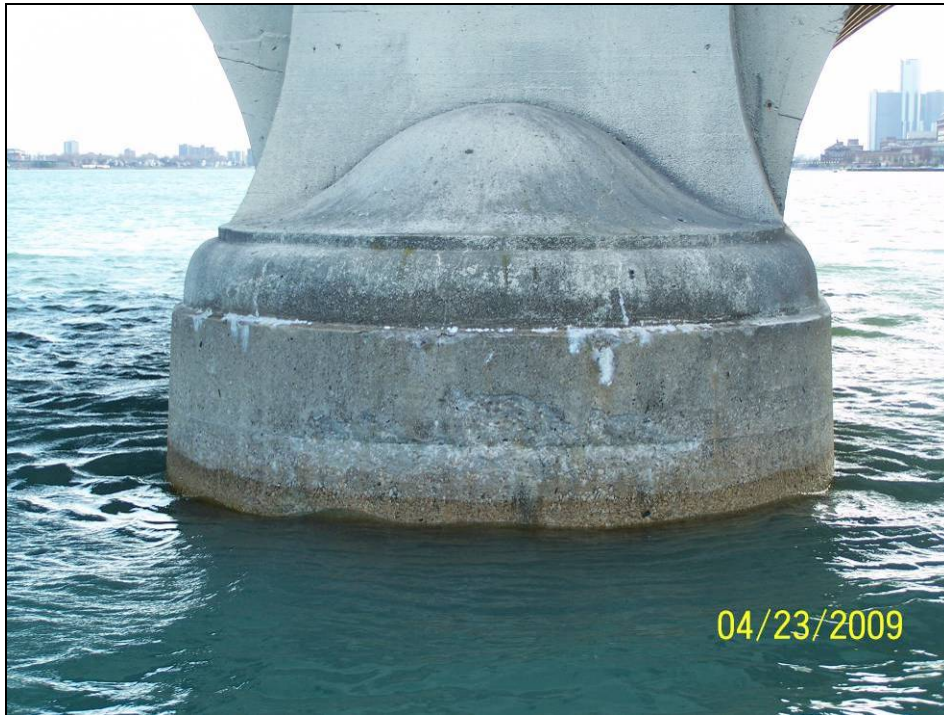
Photograph 41. View of Pier 9 Upstream Nose.
