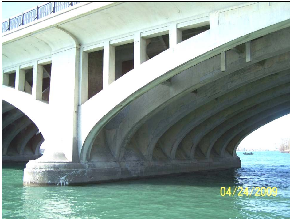
Photograph 7. View of Pier 1 North Face.
