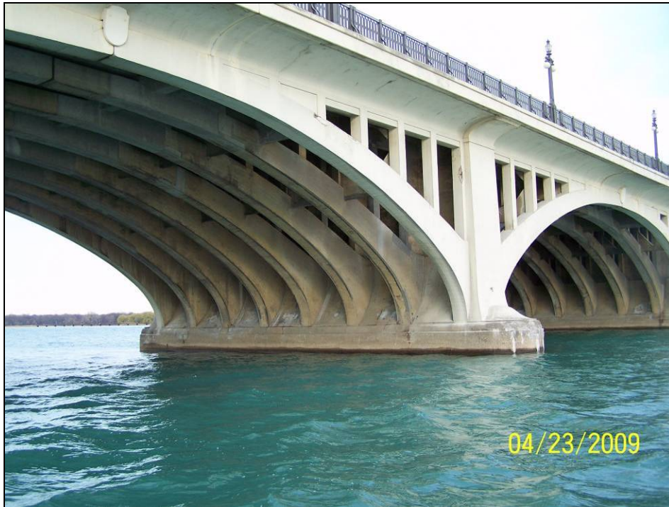
Photograph 35. View of Pier 8 North Face.
