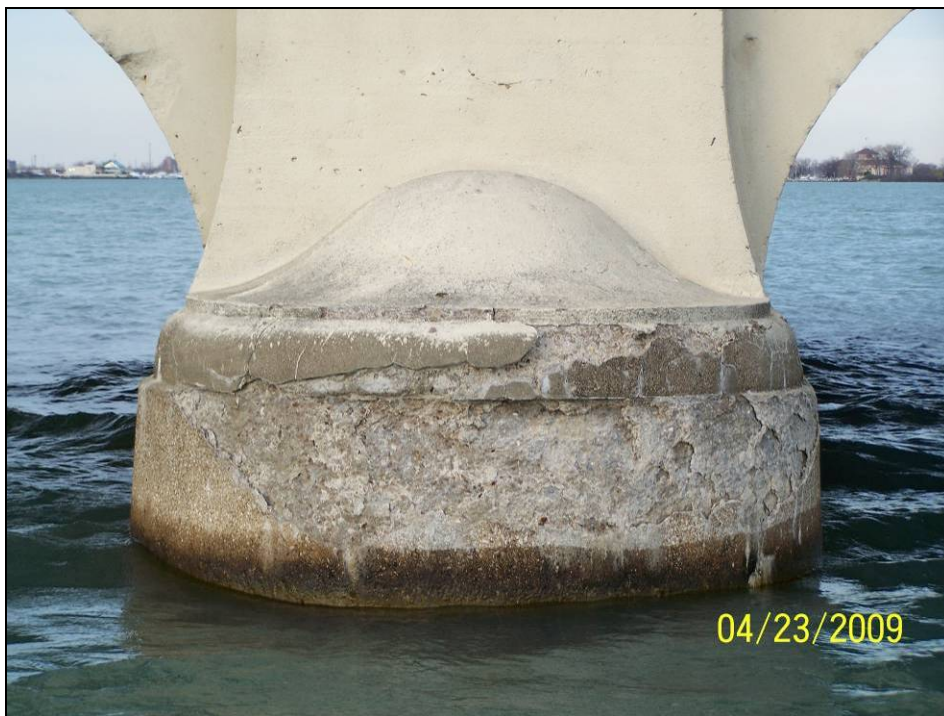
Photograph 62. View of Pier 14 Downstream Nose.
