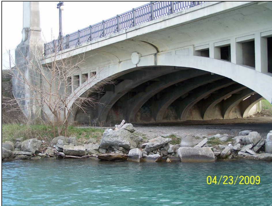
Photograph 79: View of South Abutment, North Face and East Face.
